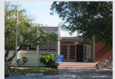
May Sands School Window/Door Replacements
