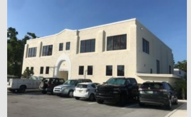
Old Gymnasium Building Renovation
