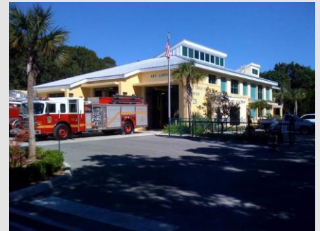
North Key Largo Fire Station
