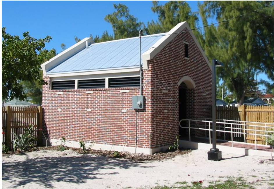
Work included re-roofing structure, and structure stabilization of vaults, arches, and brickwork.
