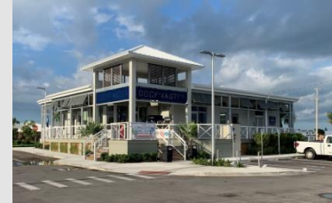
Dock Master Building
