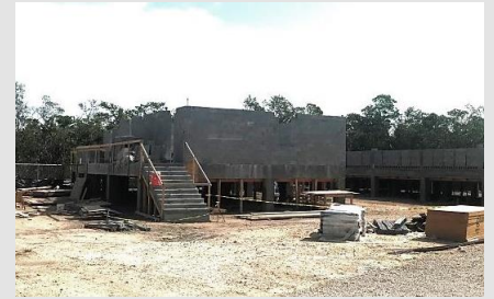
Catholic Charities Under Construction
