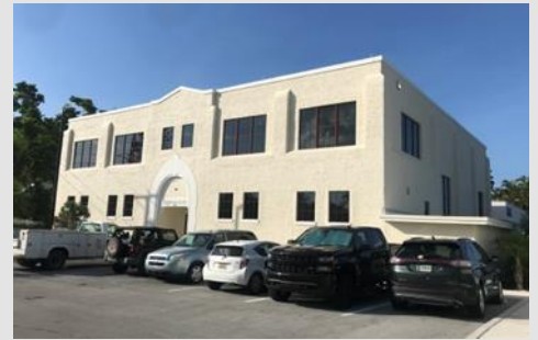
Old Gymnasium Building Renovation
