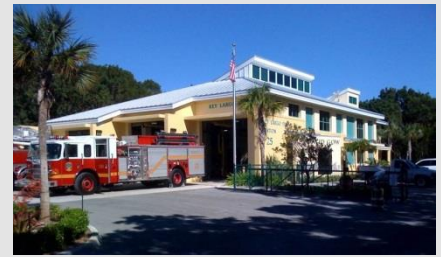
North Key Largo Fire Station
