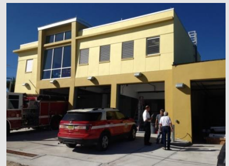
Conch Key Fire Station
