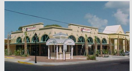
Simonton Row, 120 Simonton St.
