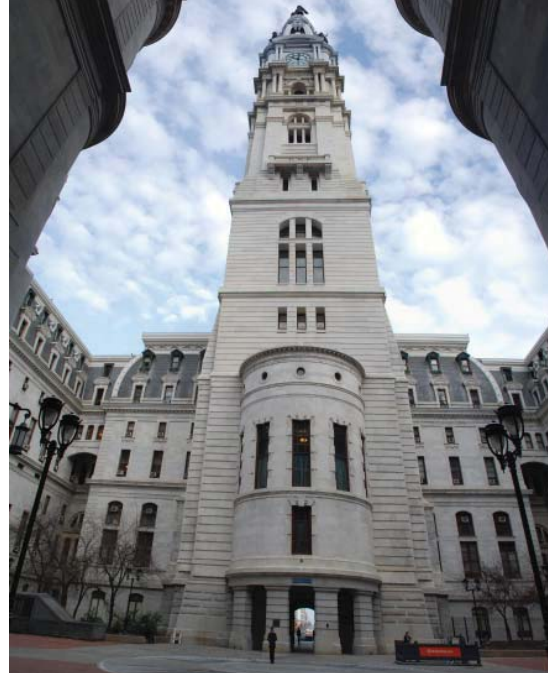
Tower after completion of masonry restoration
