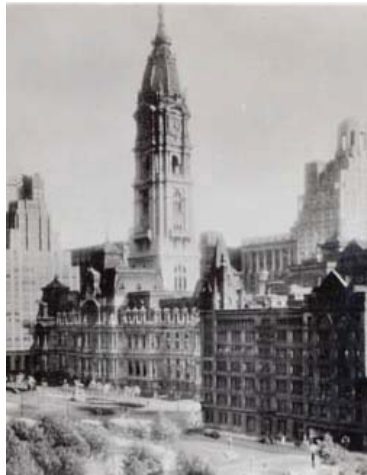
City Hall from the northwest upon completion
