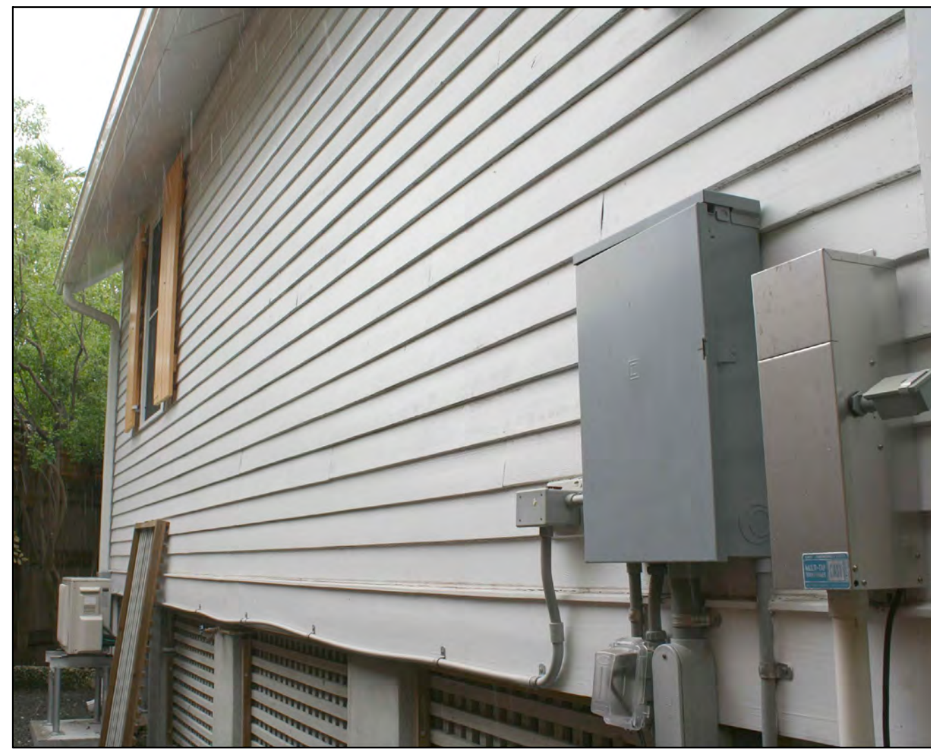
6 PHOTO DETAIL 2 (EXISTING POOL HOUSE) A2.5
