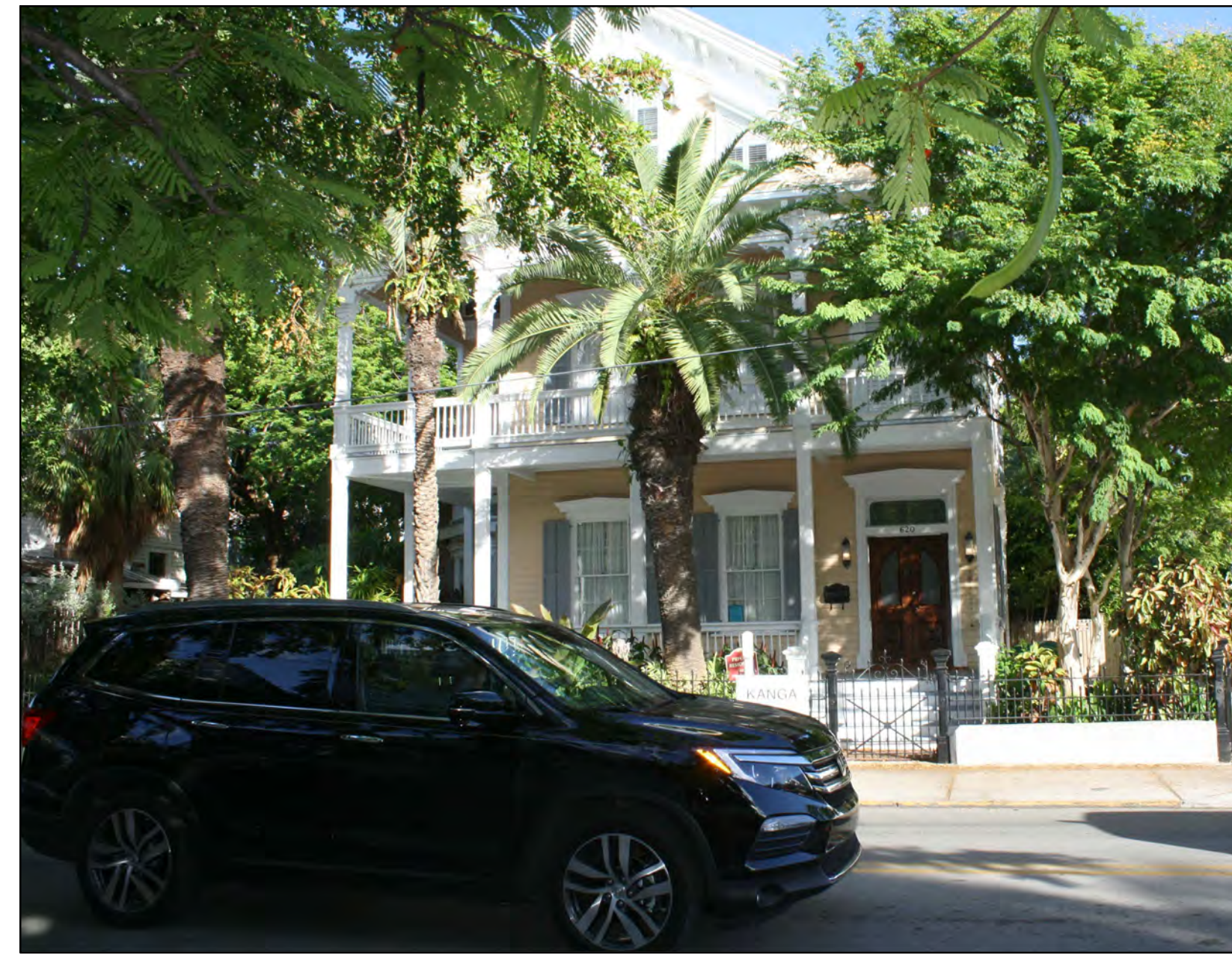
6 PHOTO DETAIL 6 (620 EATON STREET) A8.0
