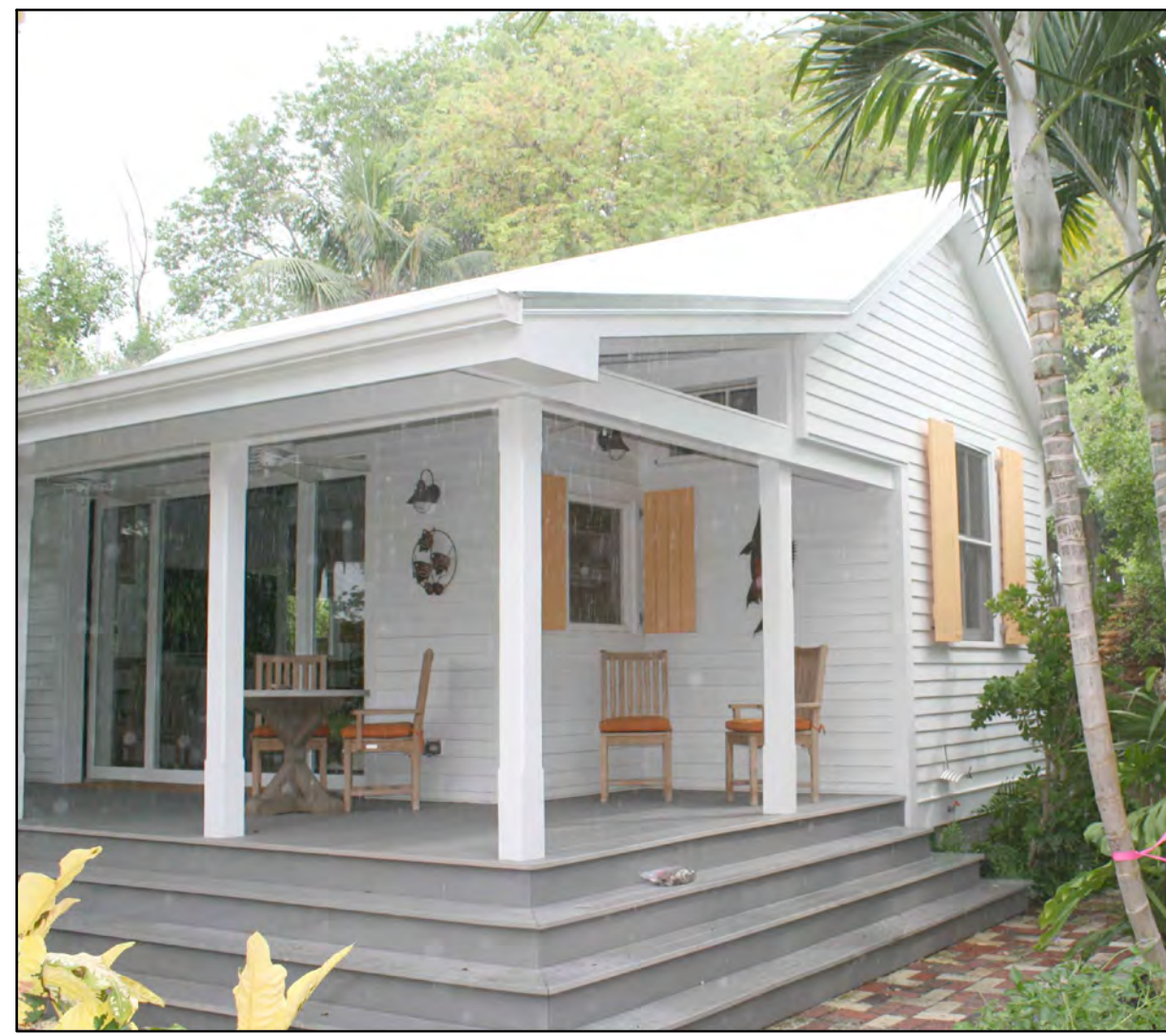
7 PHOTO DETAIL 3 (EXISTING POOL HOUSE) A2.5
