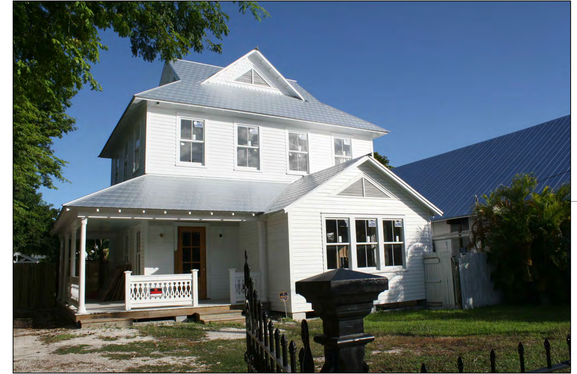
7 PHOTO DETAIL 7 (616 EATON STREET) A8.0
