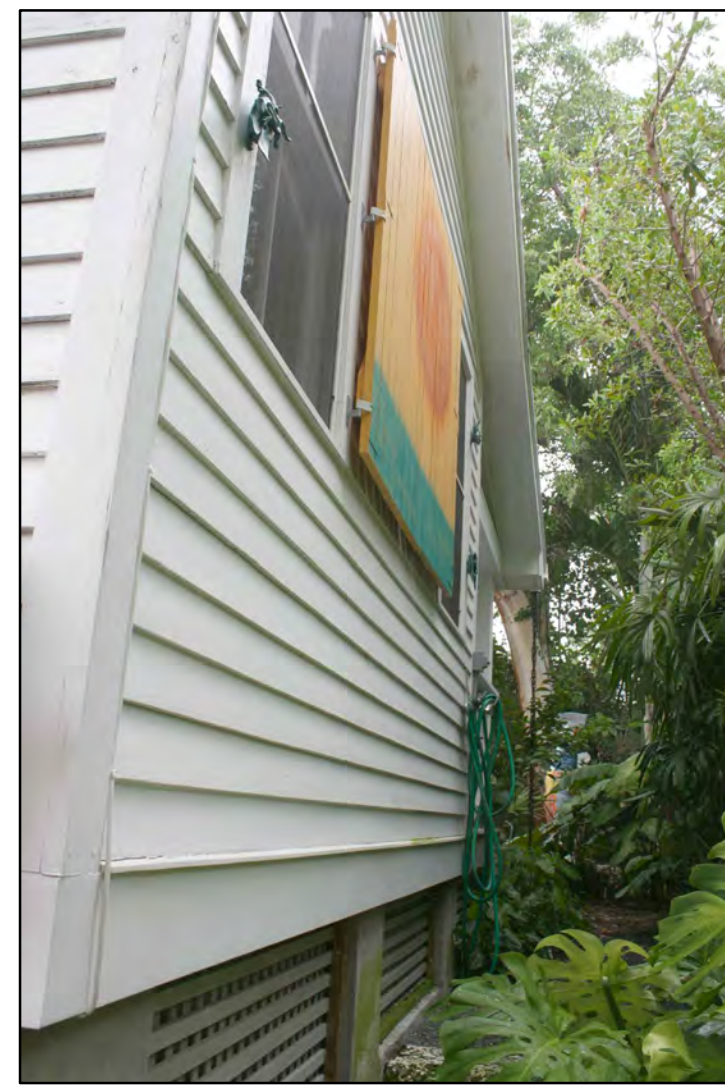
5 PHOTO DETAIL 1 (EXISTING POOL HOUSE) A2.5
