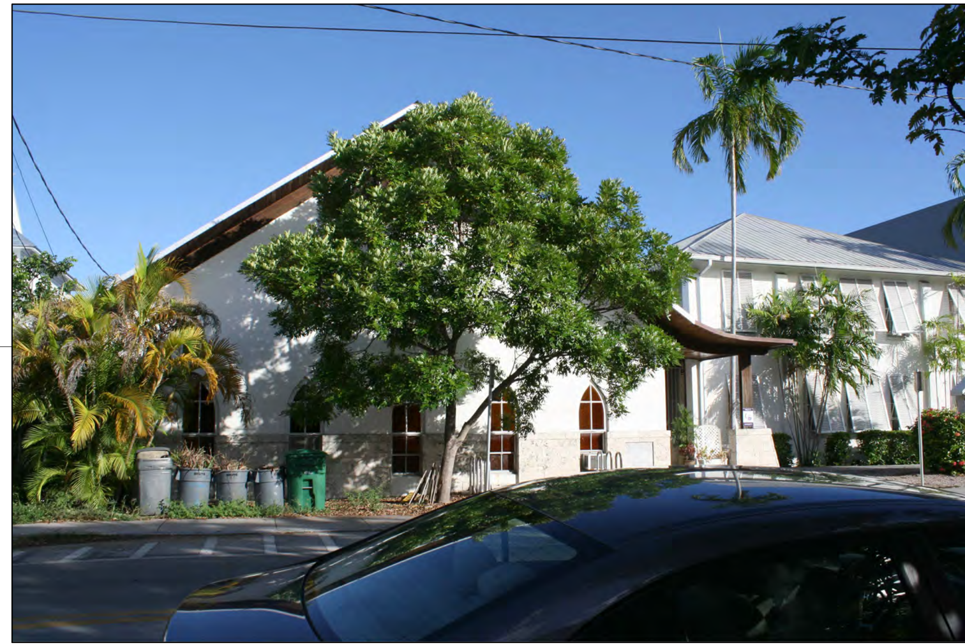
5 PHOTO DETAIL 5 (600 EATON STREET) A8.0
