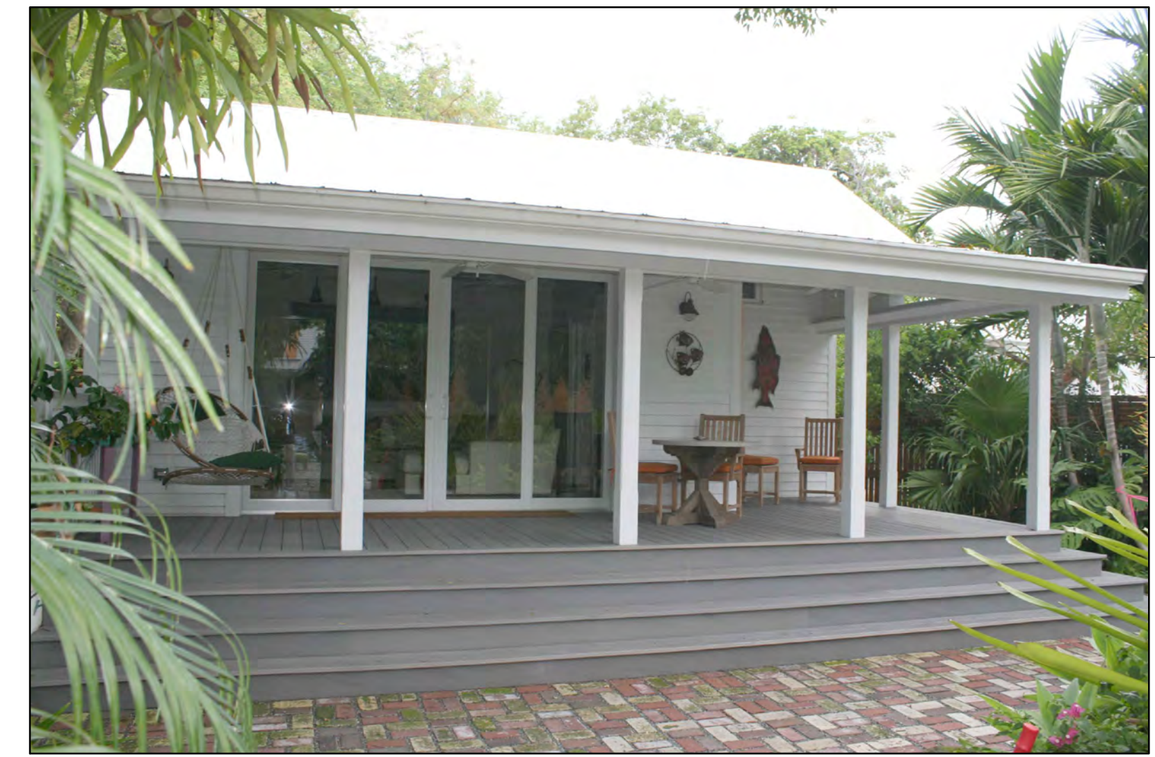
8 PHOTO DETAIL 4 (EXISTING POOL HOUSE) A2.5
