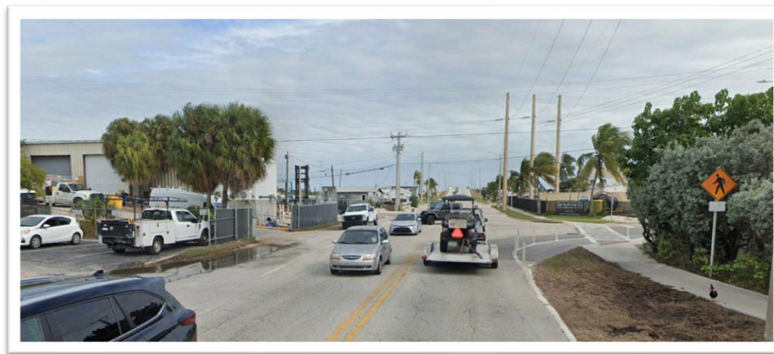
The figure shows a view of Palm Avenue approaching Eisenhower Drive, showing the two-lane configuration, driveway access to adjacent industrial and commercial properties, pedestrian crossing signage, and buffered edge areas with bollards intended to define pedestrian space and discourage encroachment.
