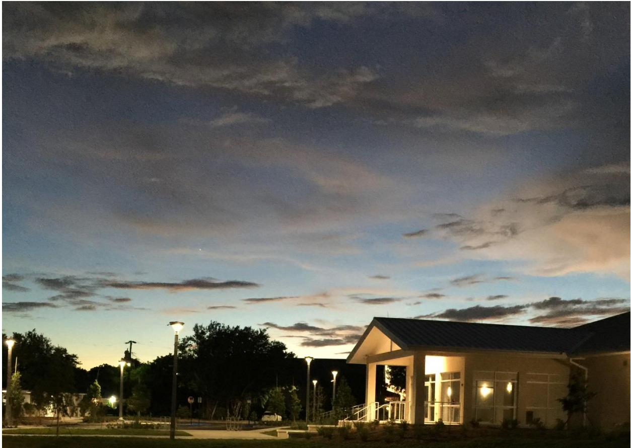
Exterior Lighting at Marathon City Hall
