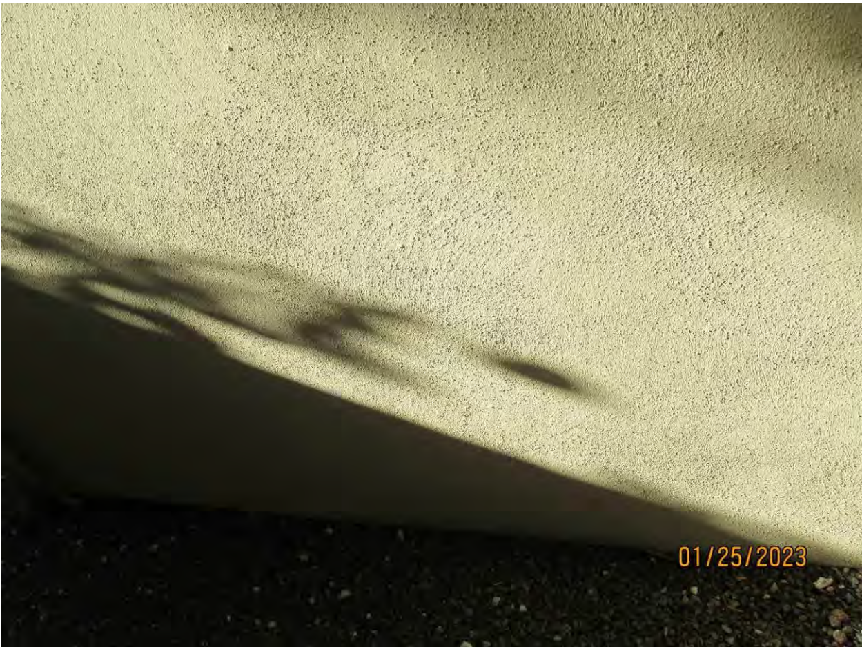
Photo of exterior wall at 915 nearest to tree-no cracks observed.
