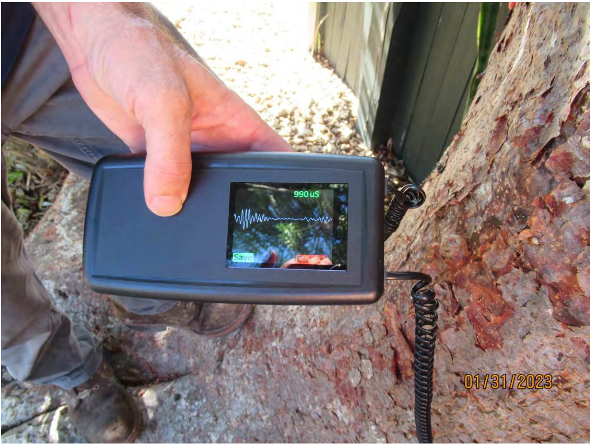
Two photos of the readings from the Tree Check Sonic Wave Tree Decay Detector showing decay in one side of the trunk.
