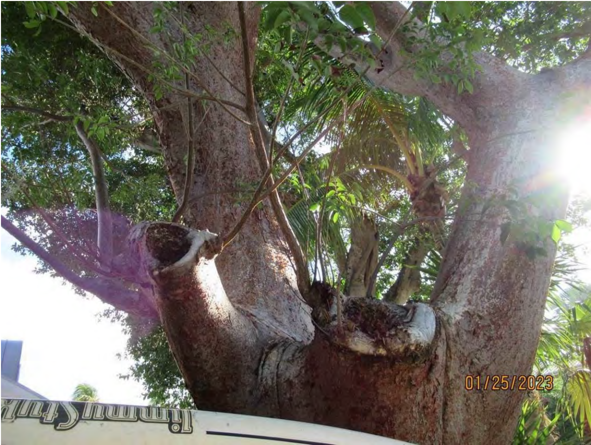
Photo of two old cut areas with decay, 915 side of tree, view 2.
