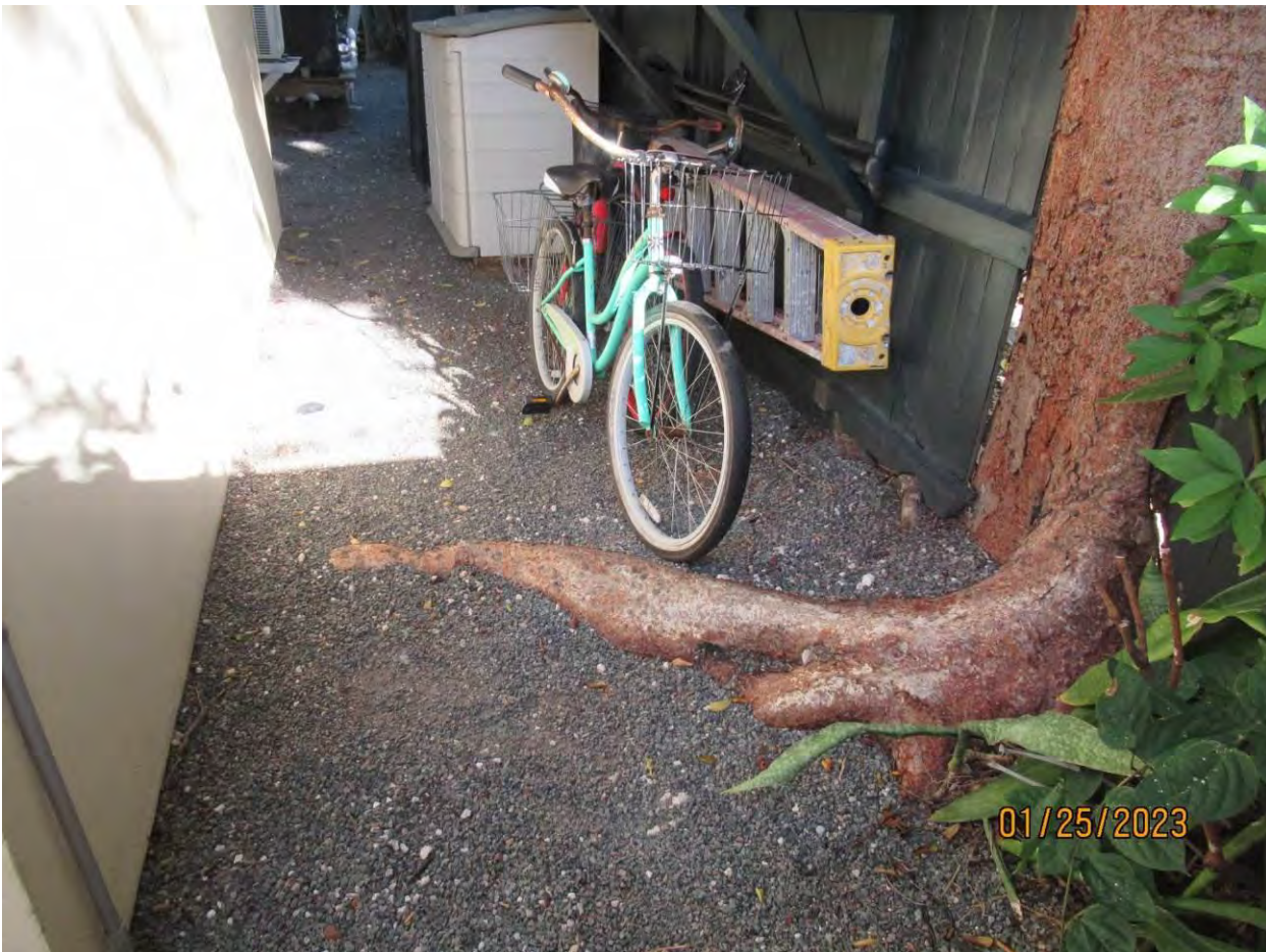
Photo of trunk and base of tree, view 1 from 915 side.
