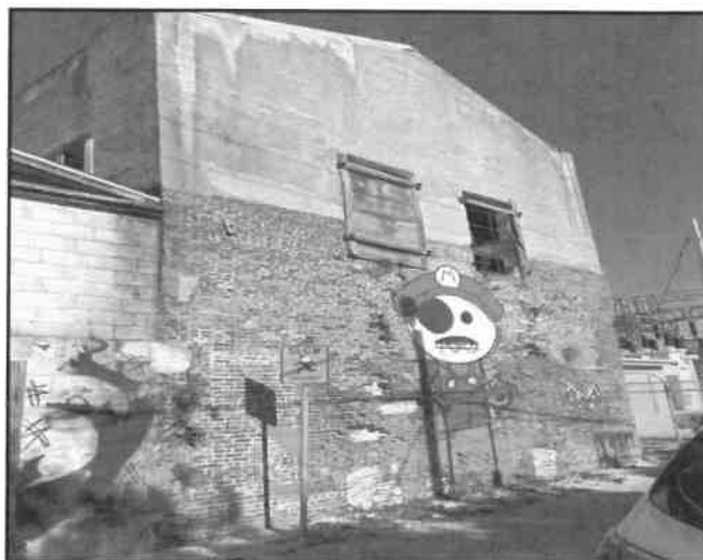
Front View of 101 Geraldine Street of Subject Property
