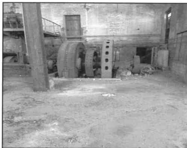
View of 100 Angela Street Building
