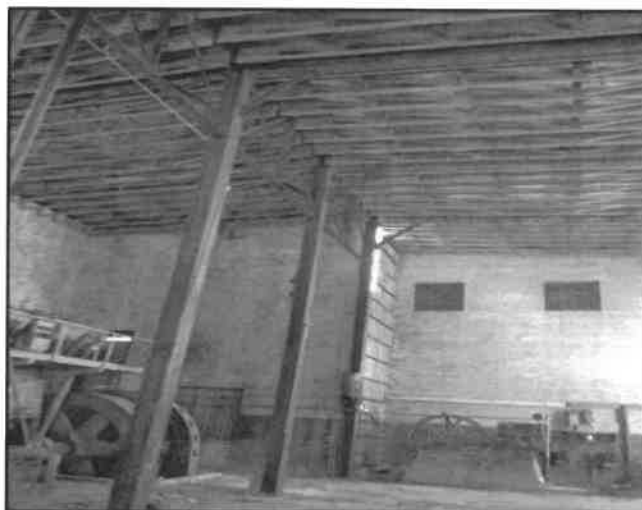
View of 100 Angela Street Building
