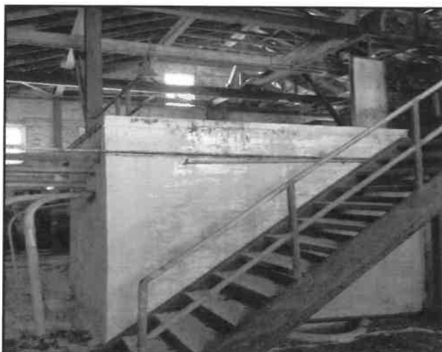
View of 709 Fort Street Building
