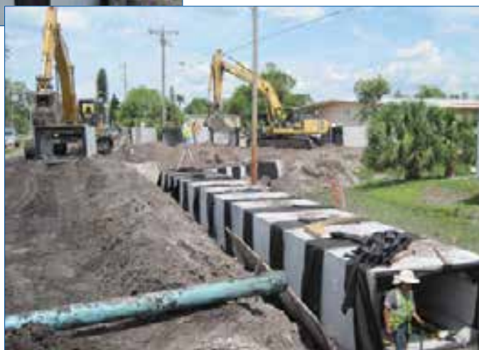
DNHI will install 262 lf of a 4-foot by 6-foot box culvert as part of the Immokalee stormwater improvements.
