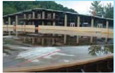
CDM Smith provided design services for replacing the the South Park Ice Rink's slab, cooling grid, dasher boards, and adjacent concrete.
