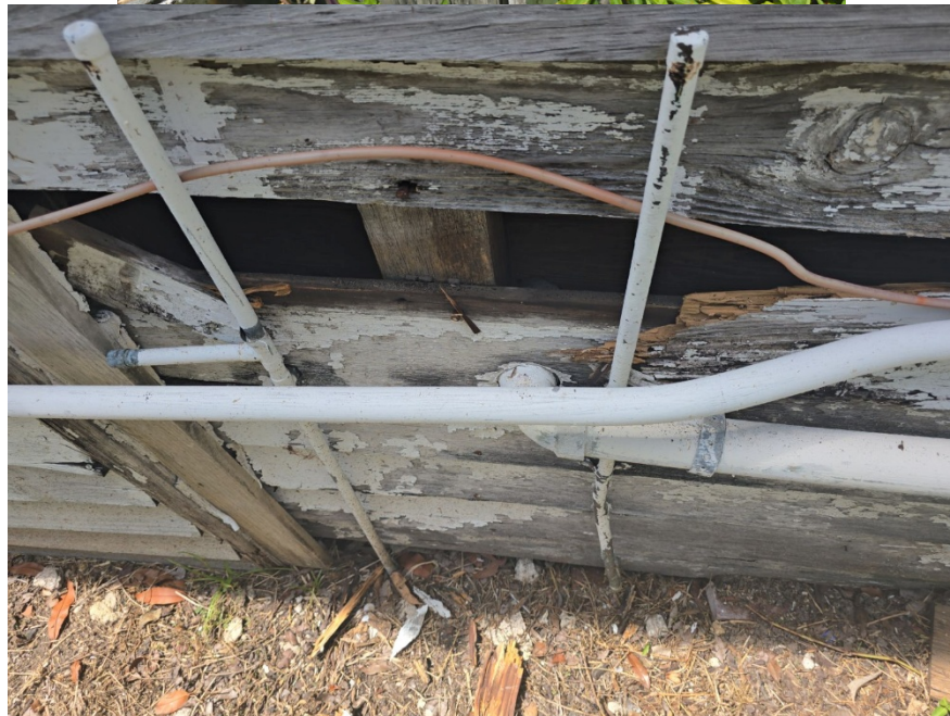
CONDITION OF EXTERIOR SIDING
