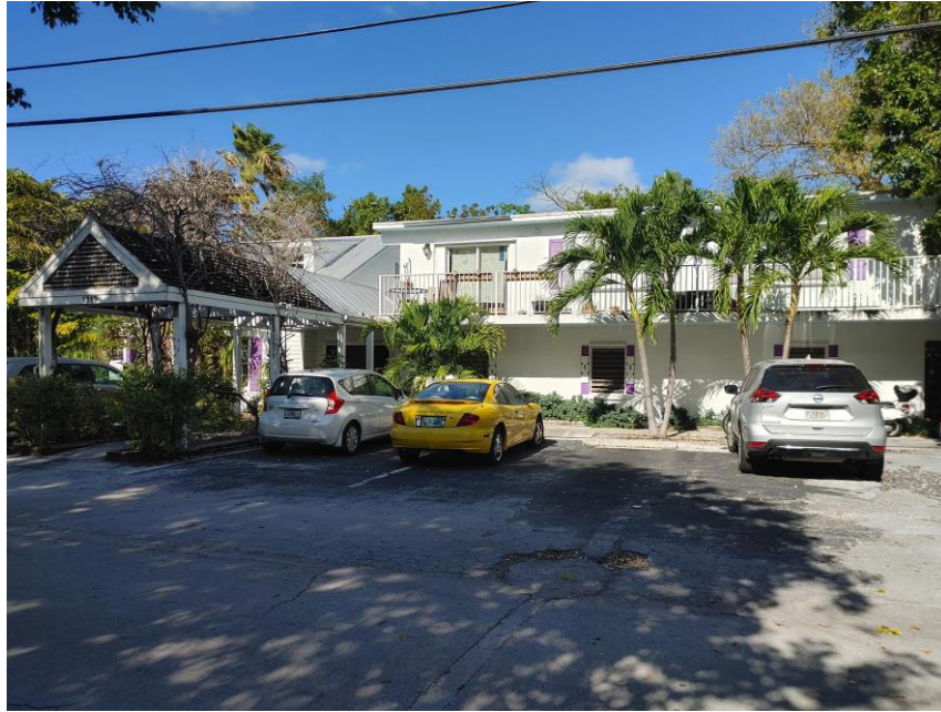
Site Visit – 1317 William Street – March 4, 2021
