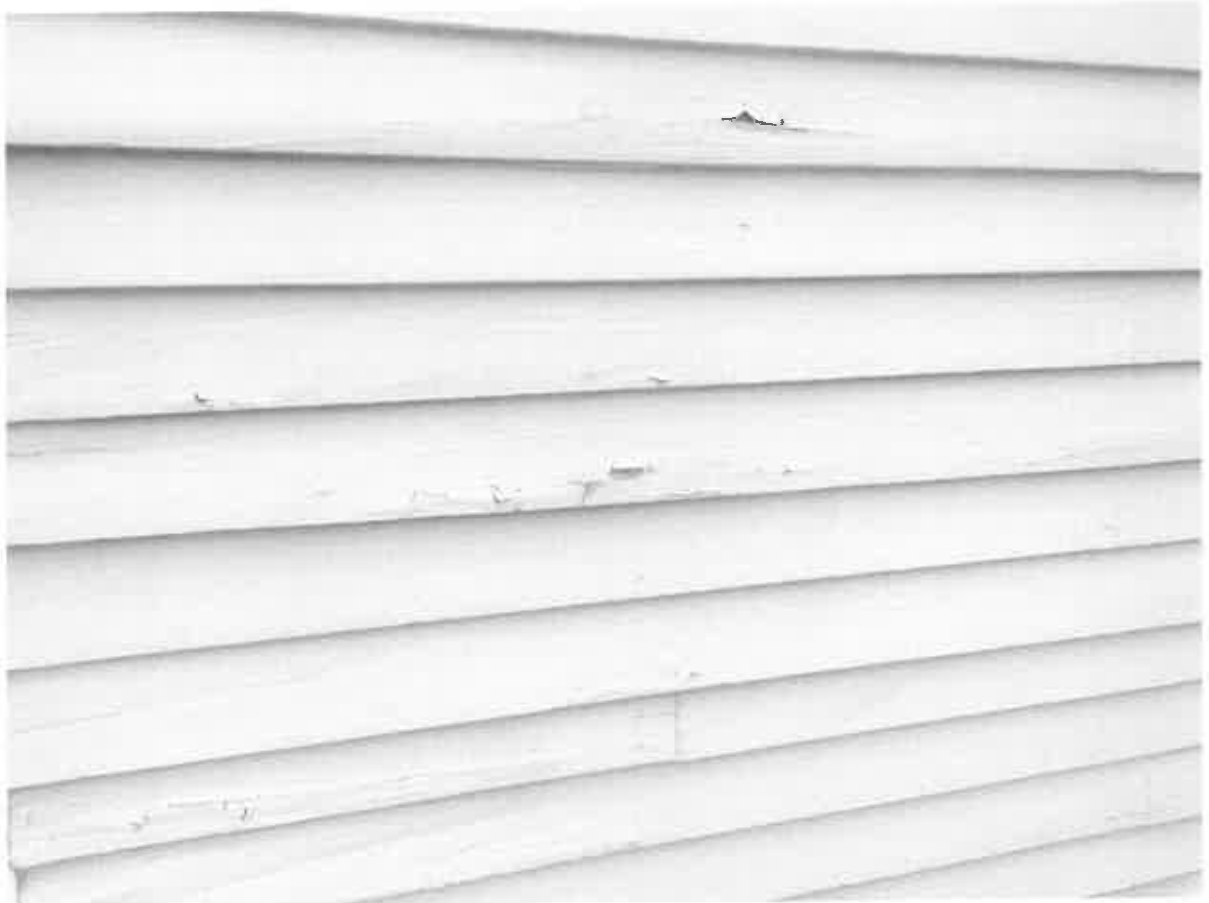
Siding cracking and peeling, also nail heads pulling out.
