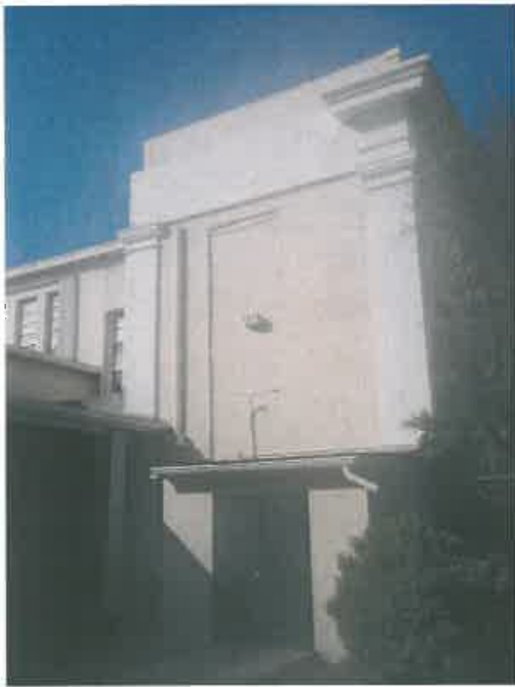
Building A, west façade. The shed at base shall be removed. All window shutters shall be removed.
