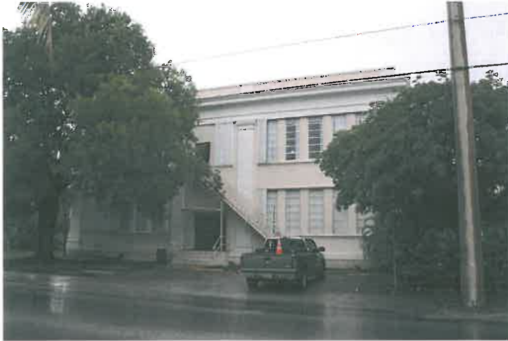
Building A, north elevation. Photo taken from across United Street. All window shutters will be removed, as well as all a/c conduit and electrical conduit. All asphalt in parking lot to be removed.
