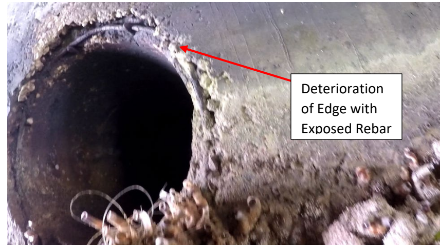
Deficiency B-88: Culvert Panel 128-129 (Station 9+43)
