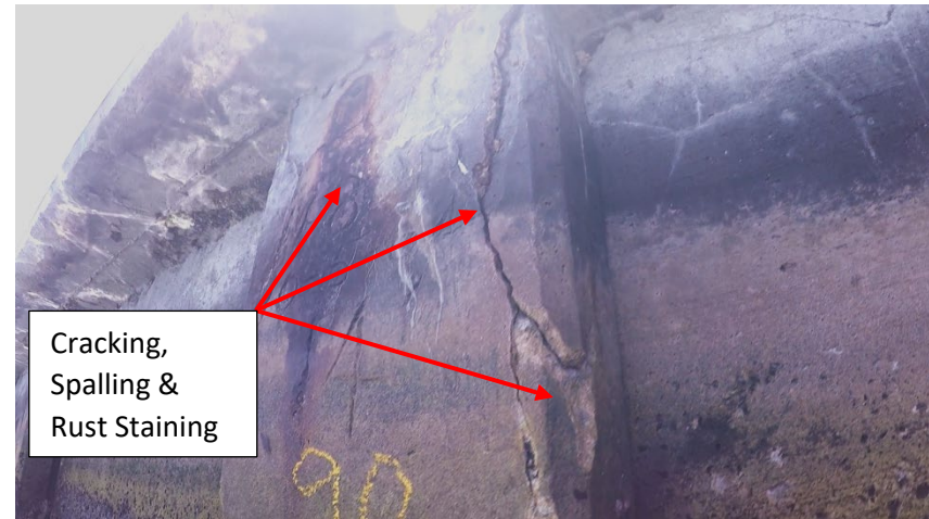
Deficiency B-93: Pile/Cap 133 (Station 9+70)
