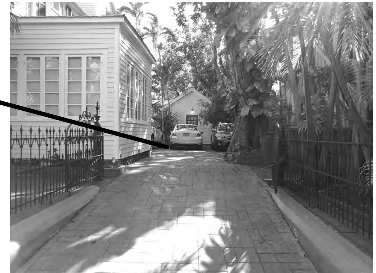
524 Simonton (accessory structure/ former garage?)
