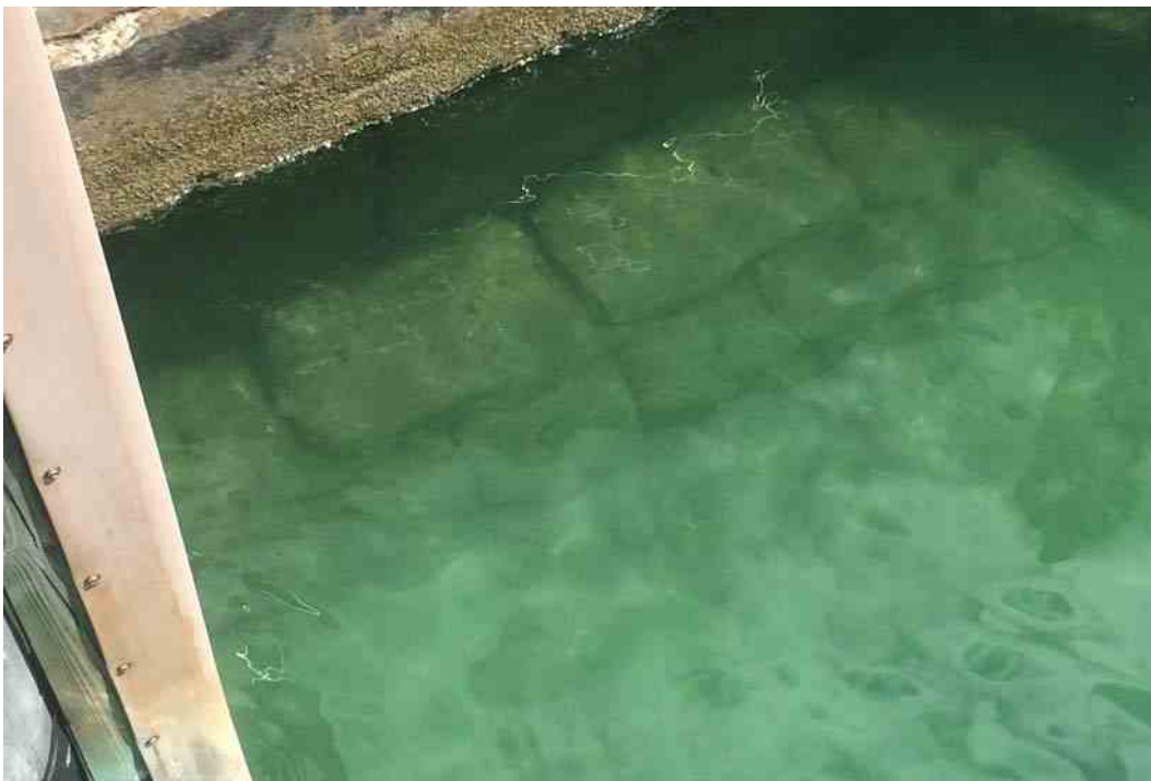
4) Sand-Cement Bags by Toe of Seawall
