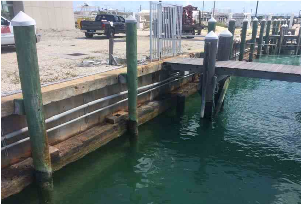
1) Typical View of Existing Seawall
