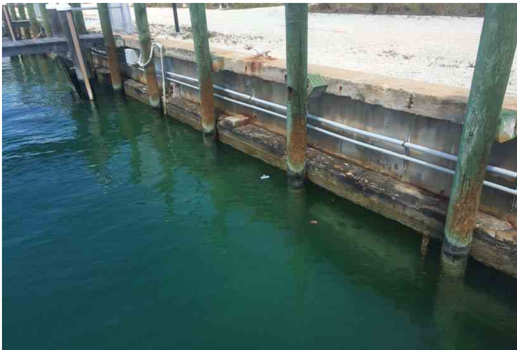
2) Typical View of Existing Seawall
