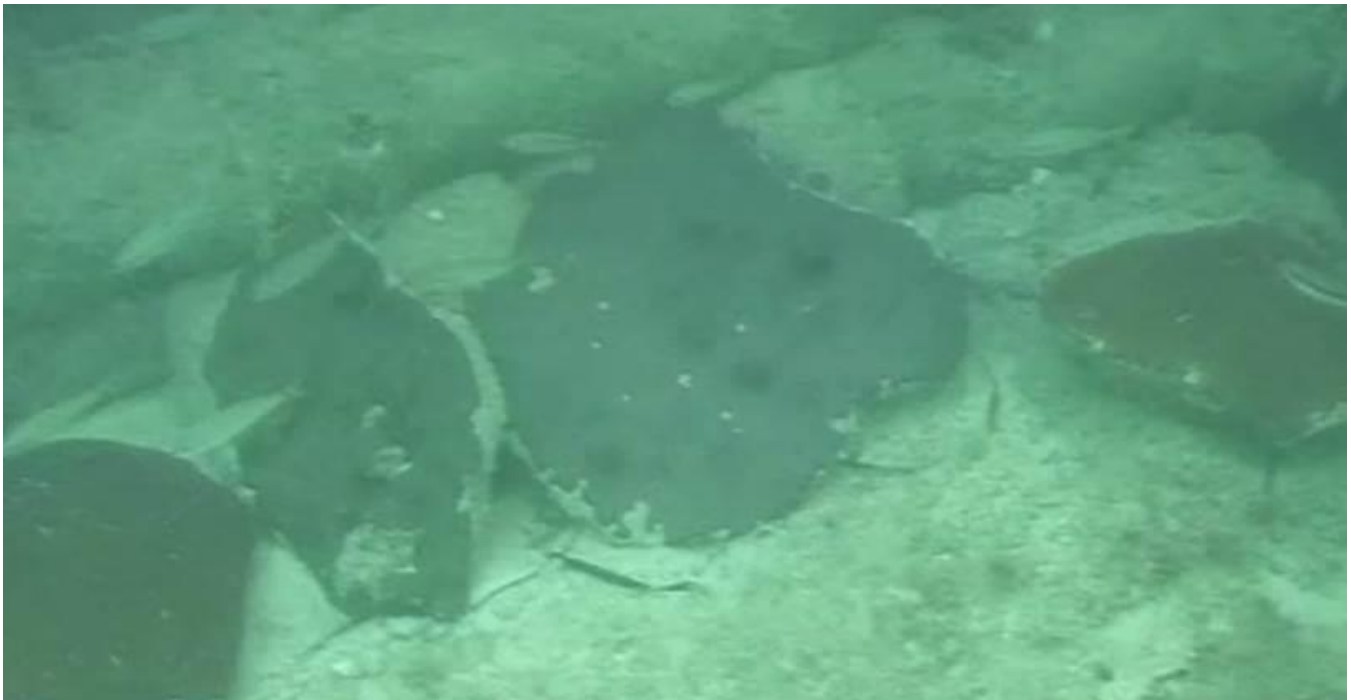
Insert 10: Toe of Existing Seawall – NOAA placed Corals
