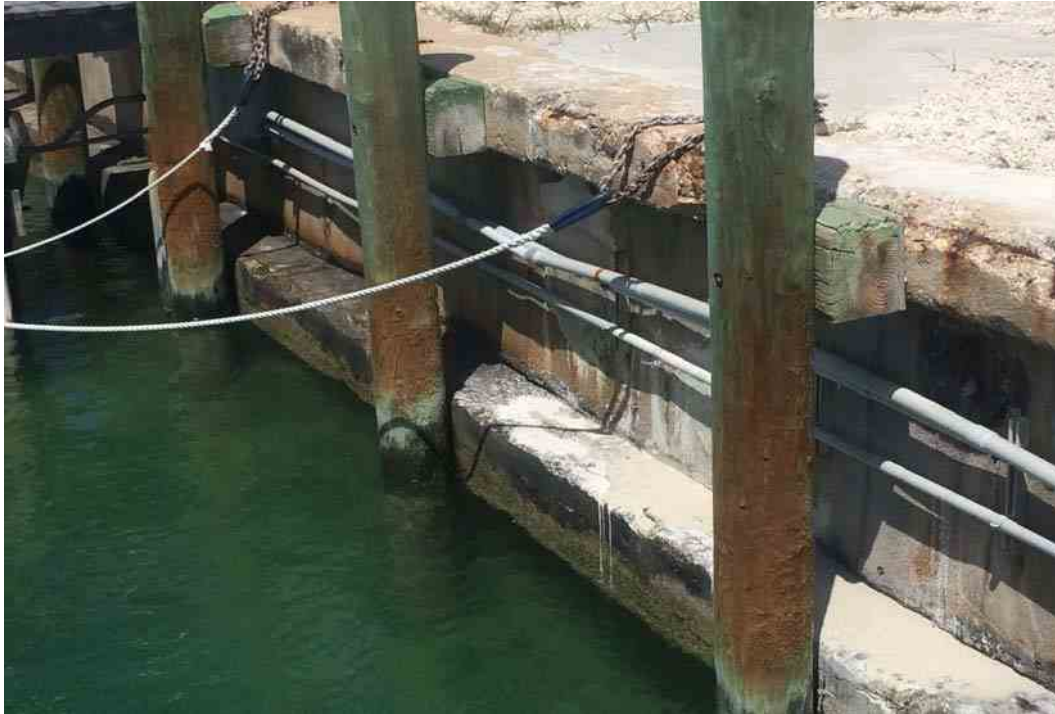
5) Close-Up View of Seawall Front
