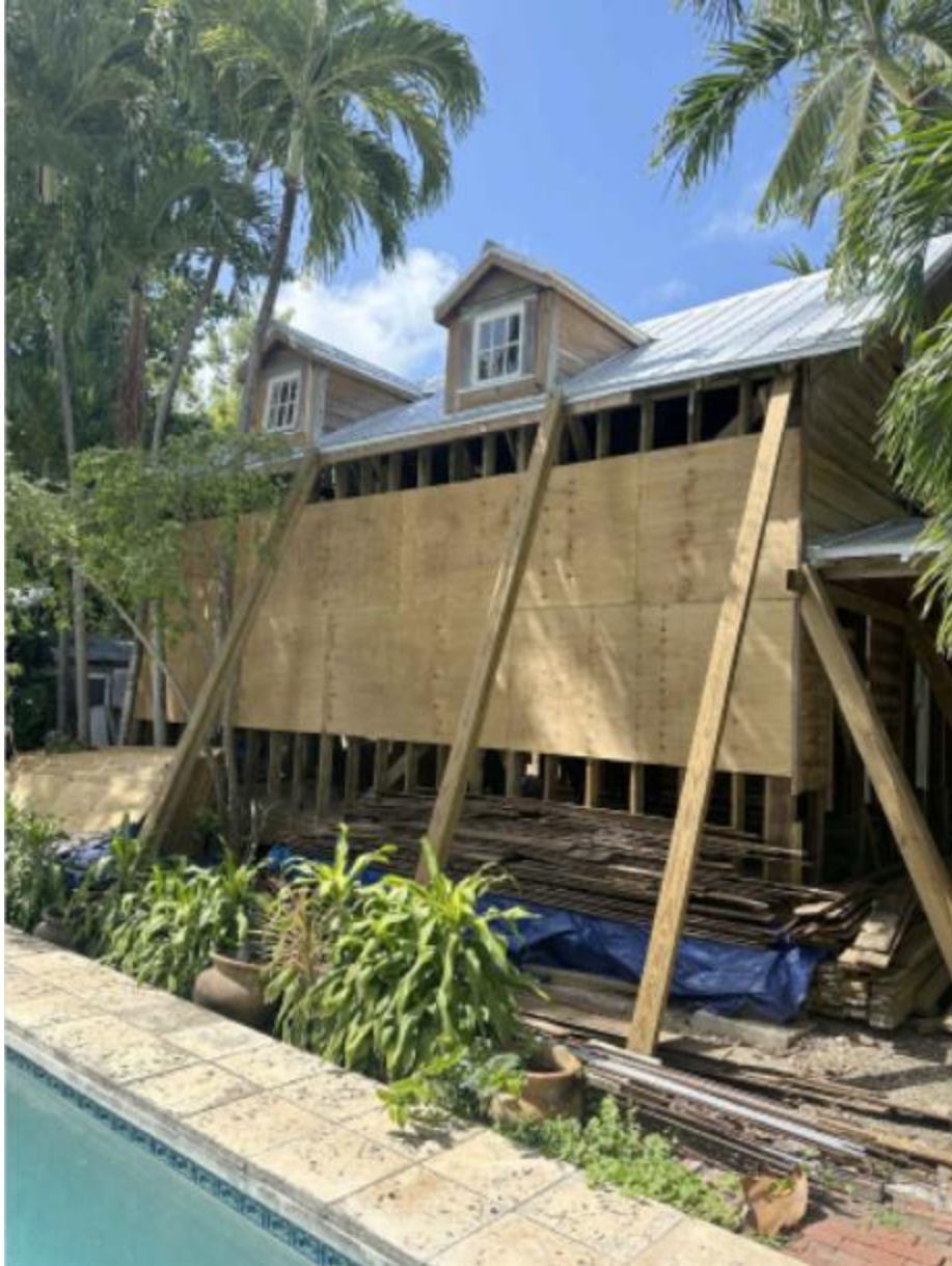
Photo of house under review after demolition.
