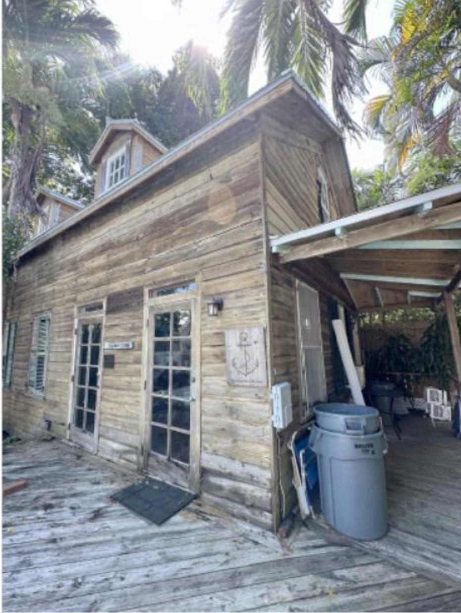
Photo of house under review before demolition.
