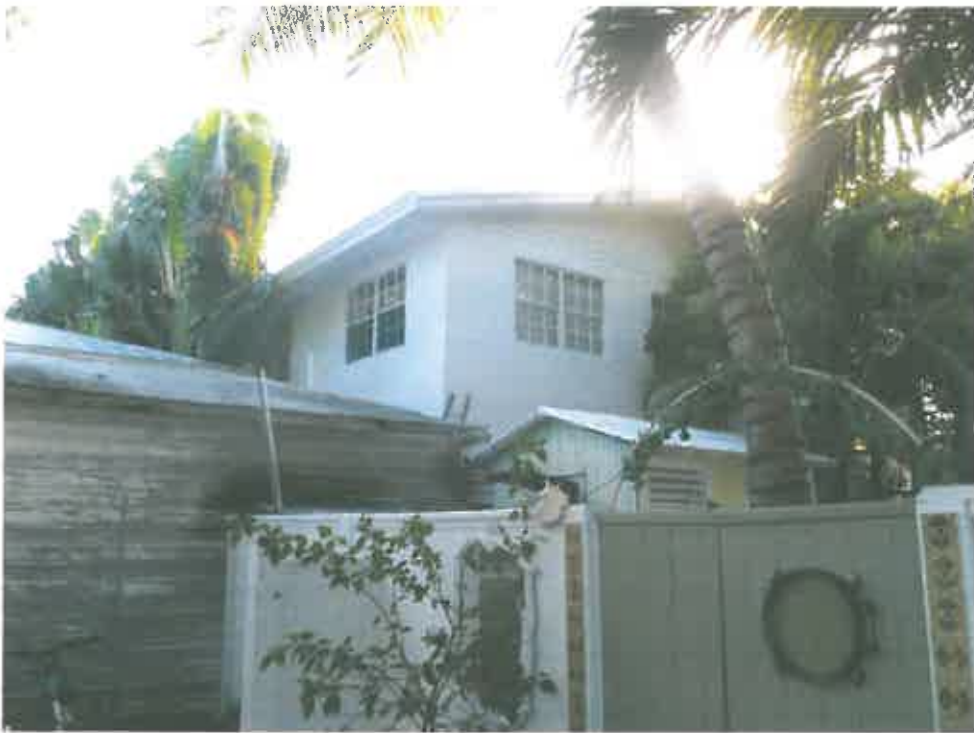
Adjacent 2 story CBS Building
