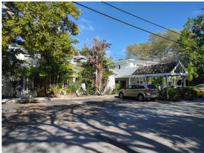
Site Visit – 1319 William Street – March 4, 2021
