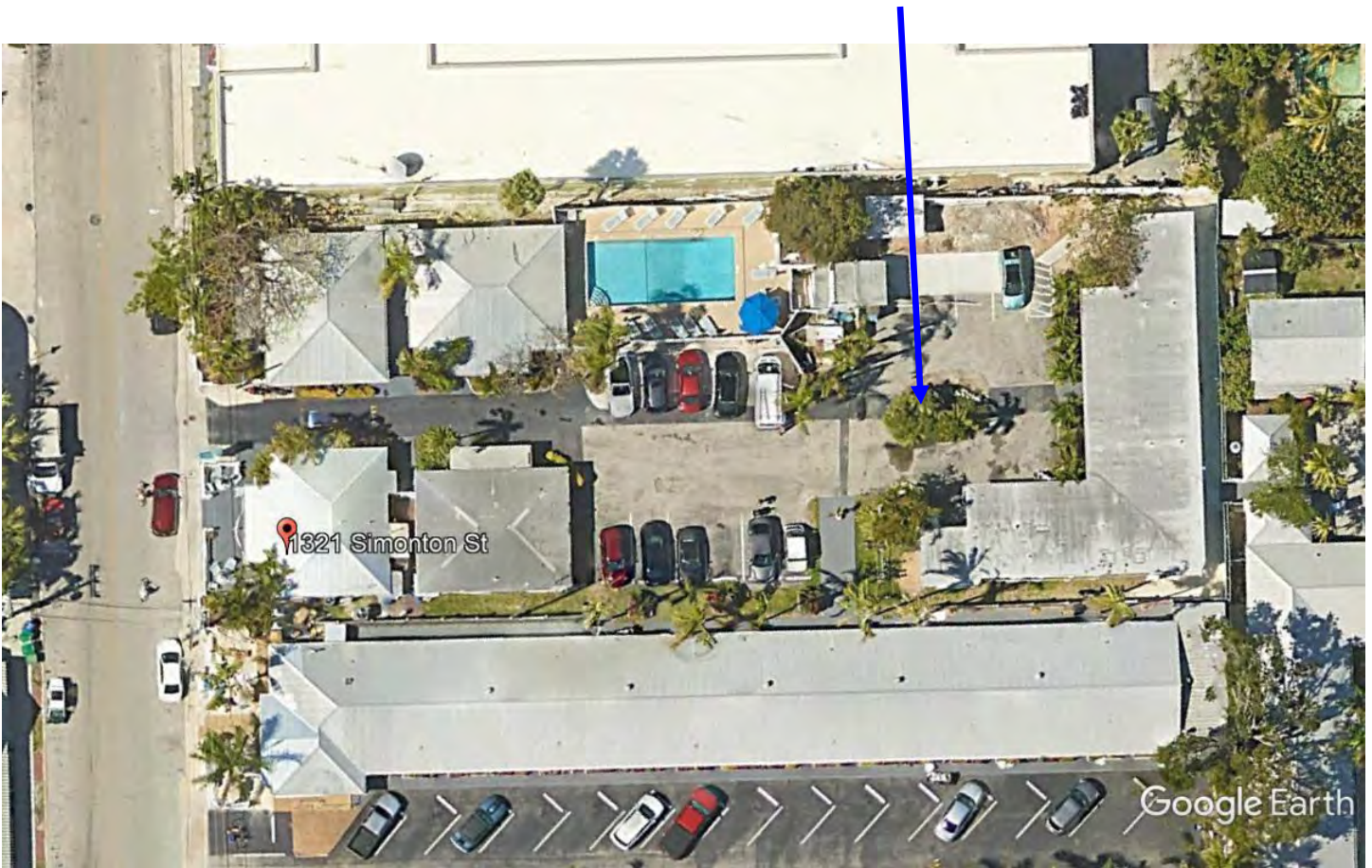
Photo showing location of tree, in parking lot planter area.
