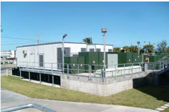
JIATF South, Emergency Generators (1.5 MW)
