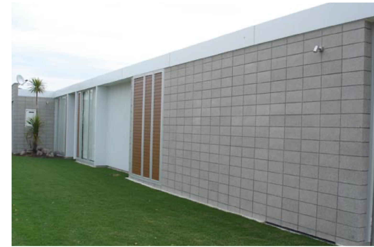
STUCCO FINISH OVER CMU - STACK BOND PATTERN
