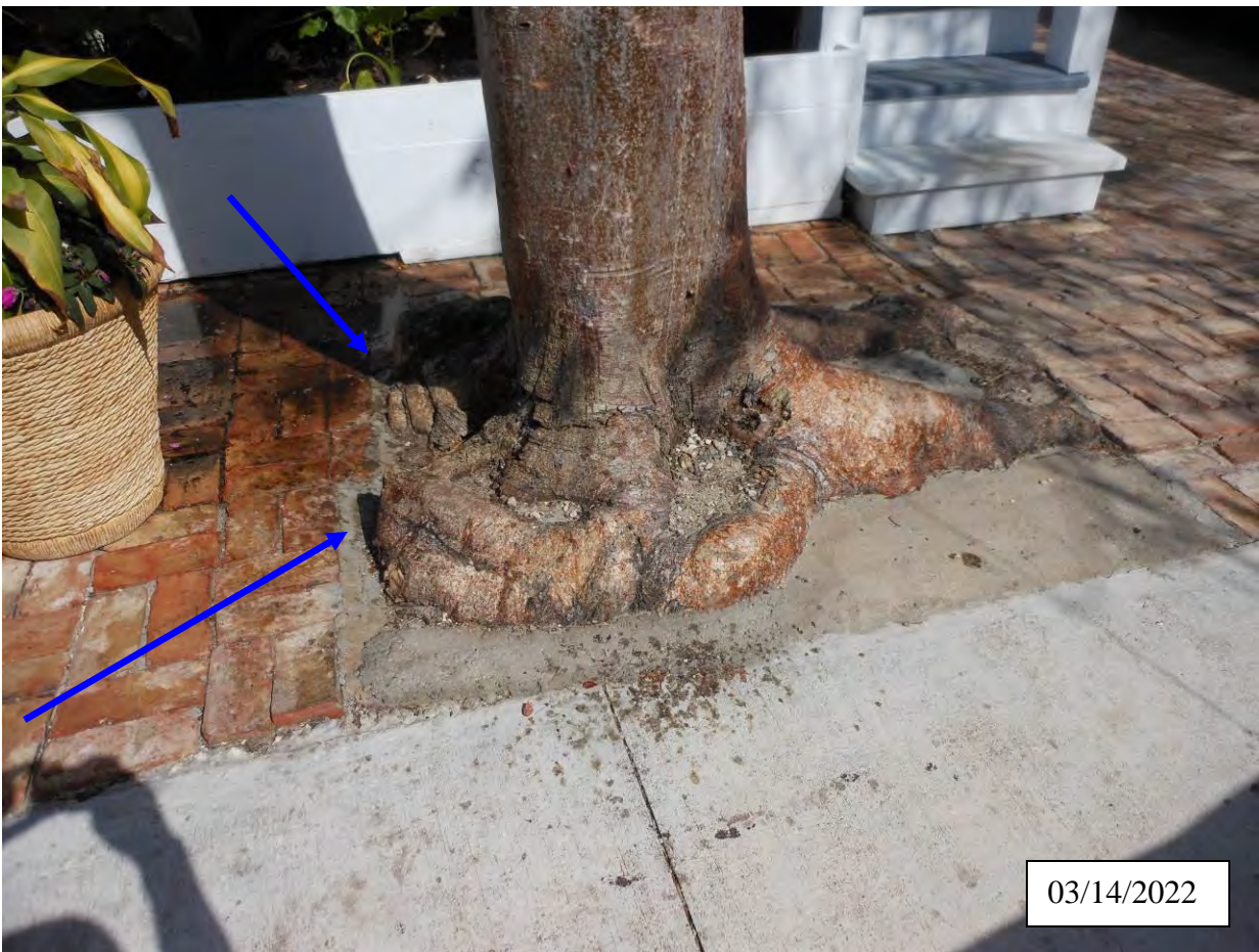
Recent photo of base of tree. Tree roots have been cut to install new pavers and concrete around tree-Tree Abuse.
