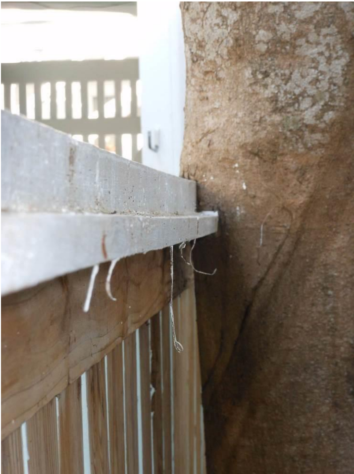
Photo showing trunk growing into deck fence, view 2.
