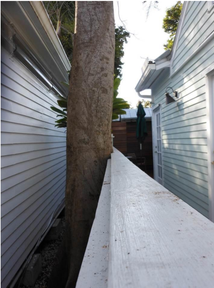
Two photos of the trunk of the tree showing trunk growing into deck fence and distance from roof eaves, view 1.
