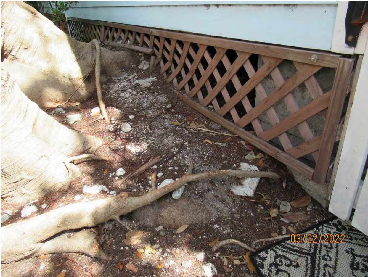
Two photos showing base of tree and roots extending under structure, view 1.
