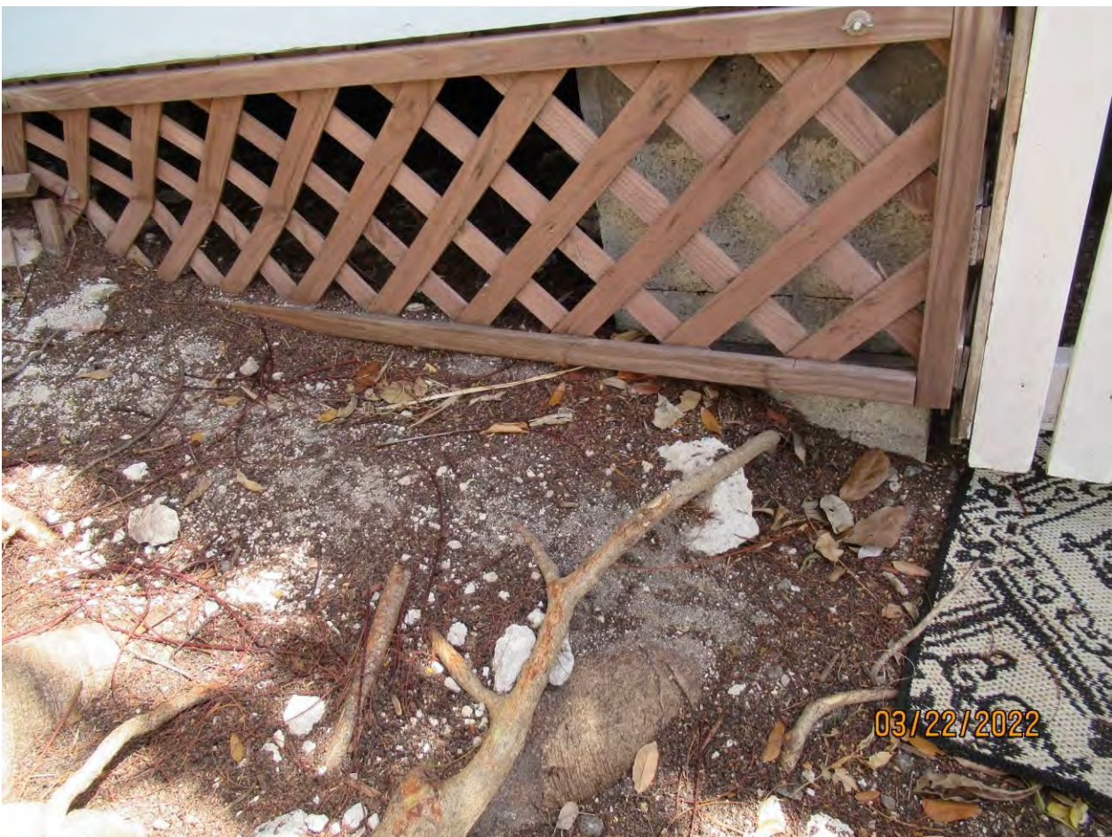
Two close up photos showing base of tree and roots extending under structure, view 1.
