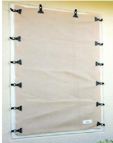
Hurricane fabric/abatement screen
