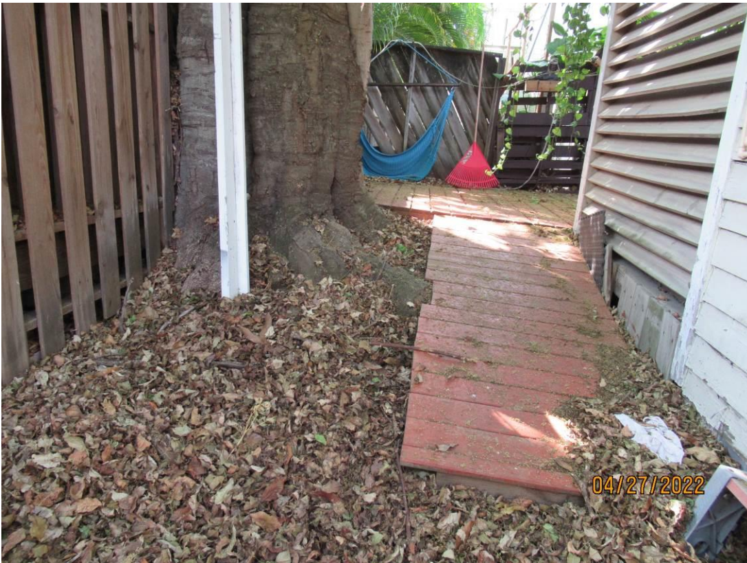
Photo showing ramp to rear deck being lifted by tree roots.
