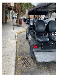
**Utilities -** The sidewalk and roadway contain manhole lids and grates with some valve box lids. Summit will make sure these are all adjusted to meet the new grade of the sidewalk and roadway. We realize the importance of not having a tripping hazard on the sidewalks and will verify compliance with the plans and standards.
