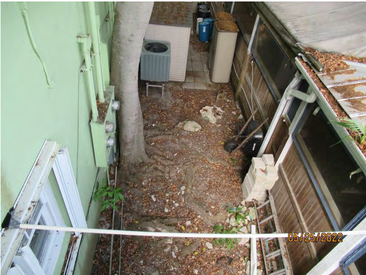
Photo showing base of tree and trunk against structure, view 2.
