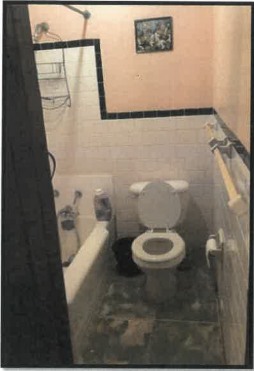
Unit 9 Lockout – bathroom
