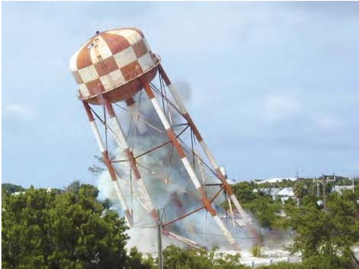
Water Tank Demolition, NAS Key West
