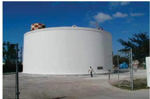
700,000 Gallon Concrete Water Tank
