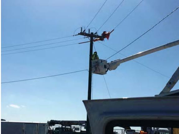
Installing Guy Wire NAS KW
