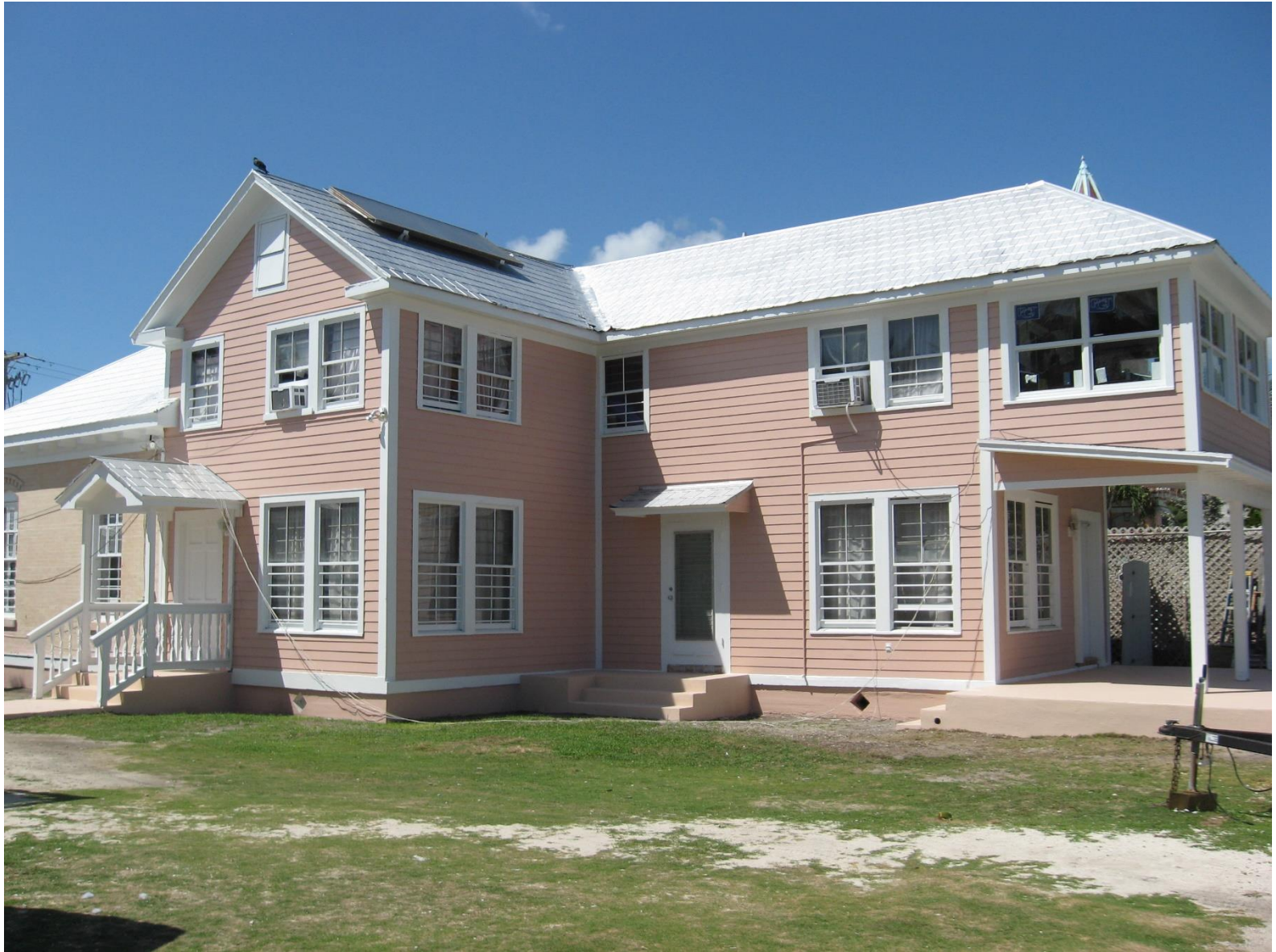
404 South Street before changing to 5 V-Crimp roofing. Notice the original masonry building to the left side.
