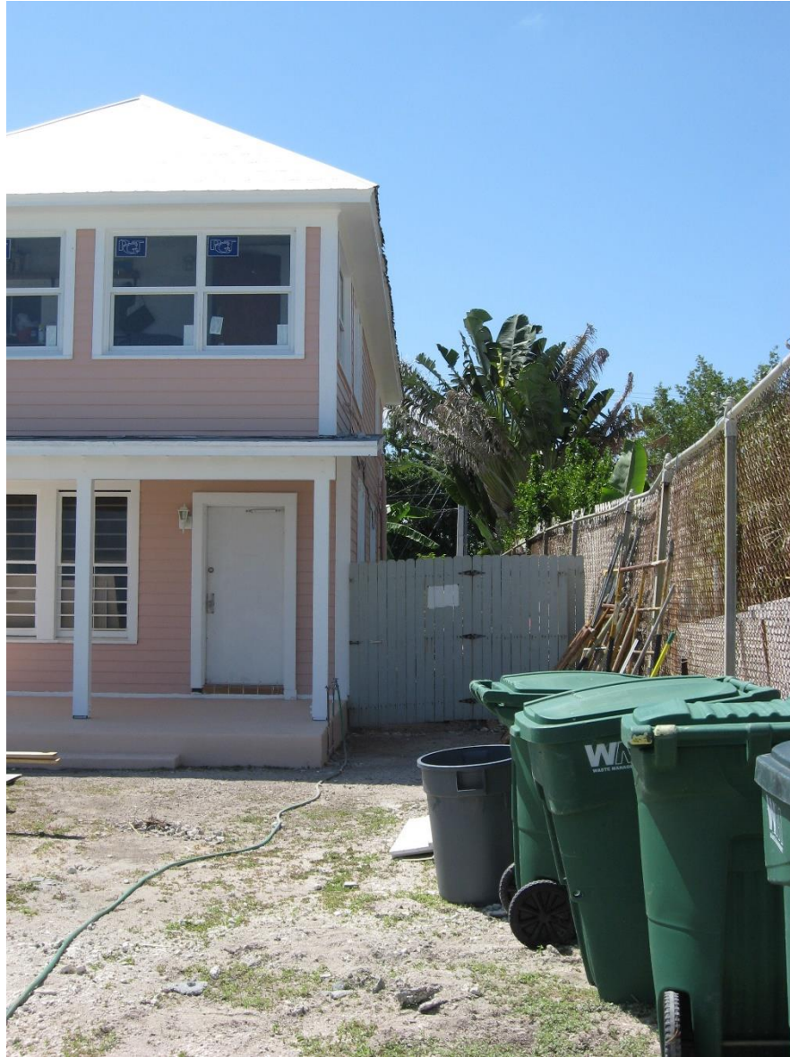
404 South Street before changing to 5 V-Crimp roofing.
