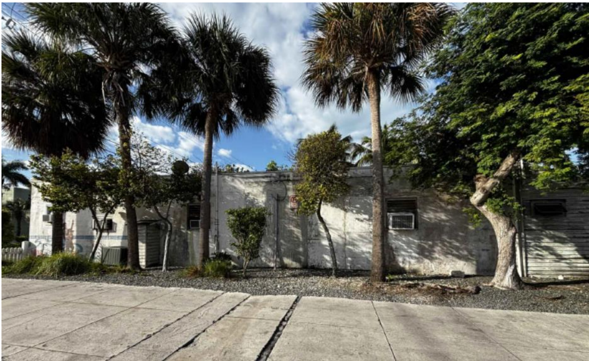
Side elevation of structure.
