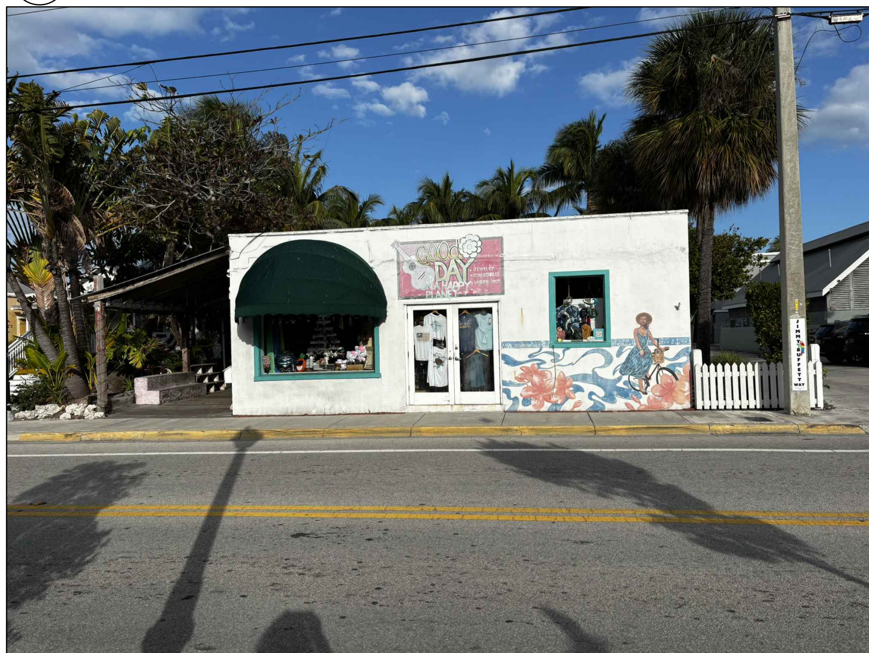
1 VIEW OF THE FRONT OF THE BUILDING (EXISTING SOUTH ELEVATION) A6 SCALE: N.T.S.
