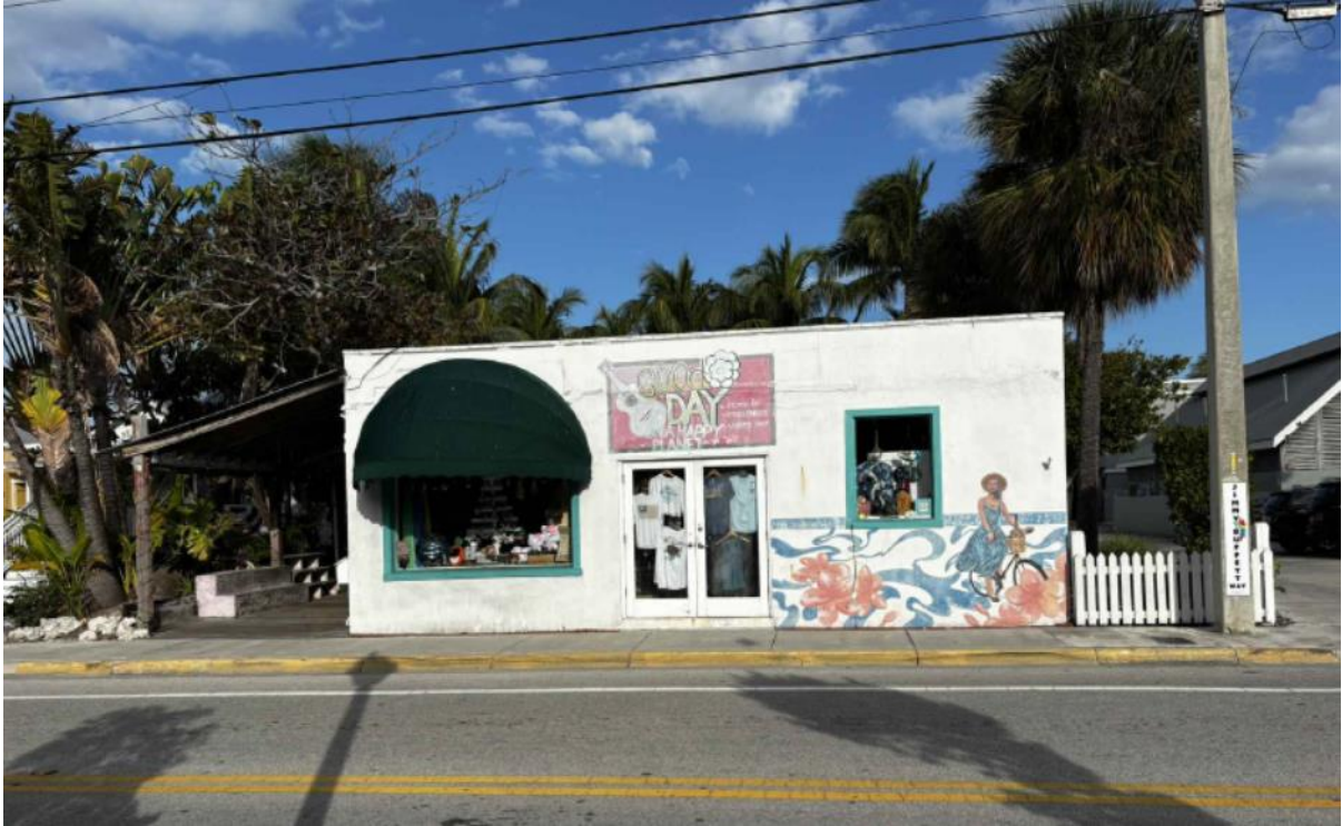
Current photo of structure.
