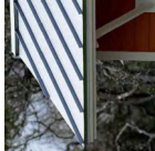
ALUMINUM ROOF PANEL OVER WOOD ROOF SYSTEM (A1)
