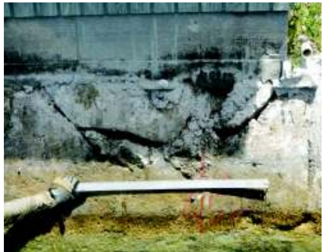
Photo 10: Spalling and cracks at Sta 65' W
