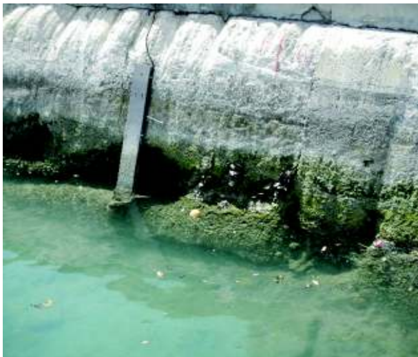
Photo 9: Cavities at waterline at Sta 15' W
