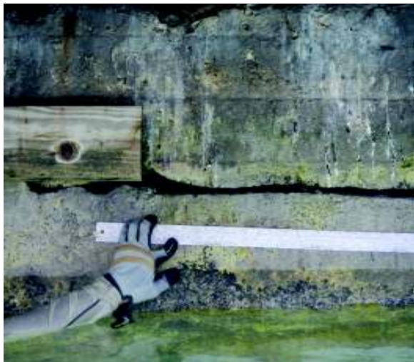
Photo 13: Cracking in wall at Sta 58' C
