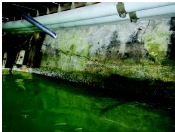
Photo 18: Cracking in wall at Sta 133' C
