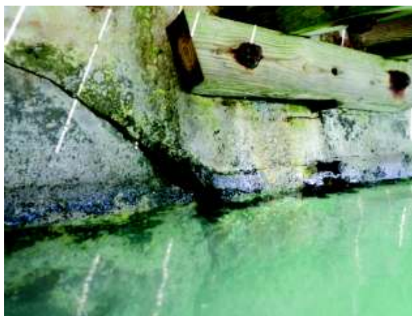
Photo 16: Cracking in wall at Sta 110' C
