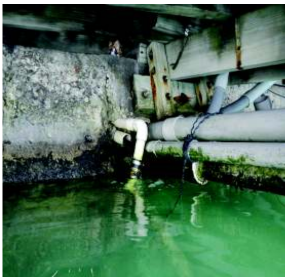
Photo 29: Utility penetrations at Sta 15' E
