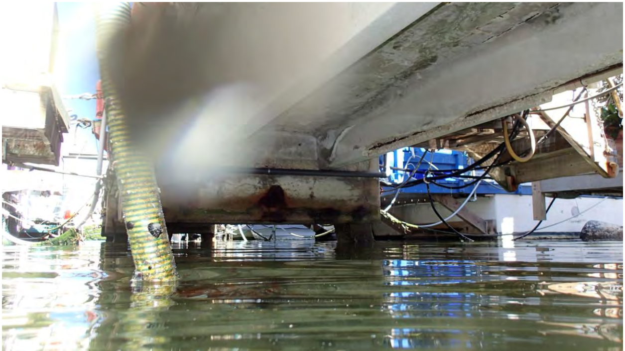
Photo of typical pier support piles showing extensive damage. Replacement of the pier is needed to prevent a structural failure.
