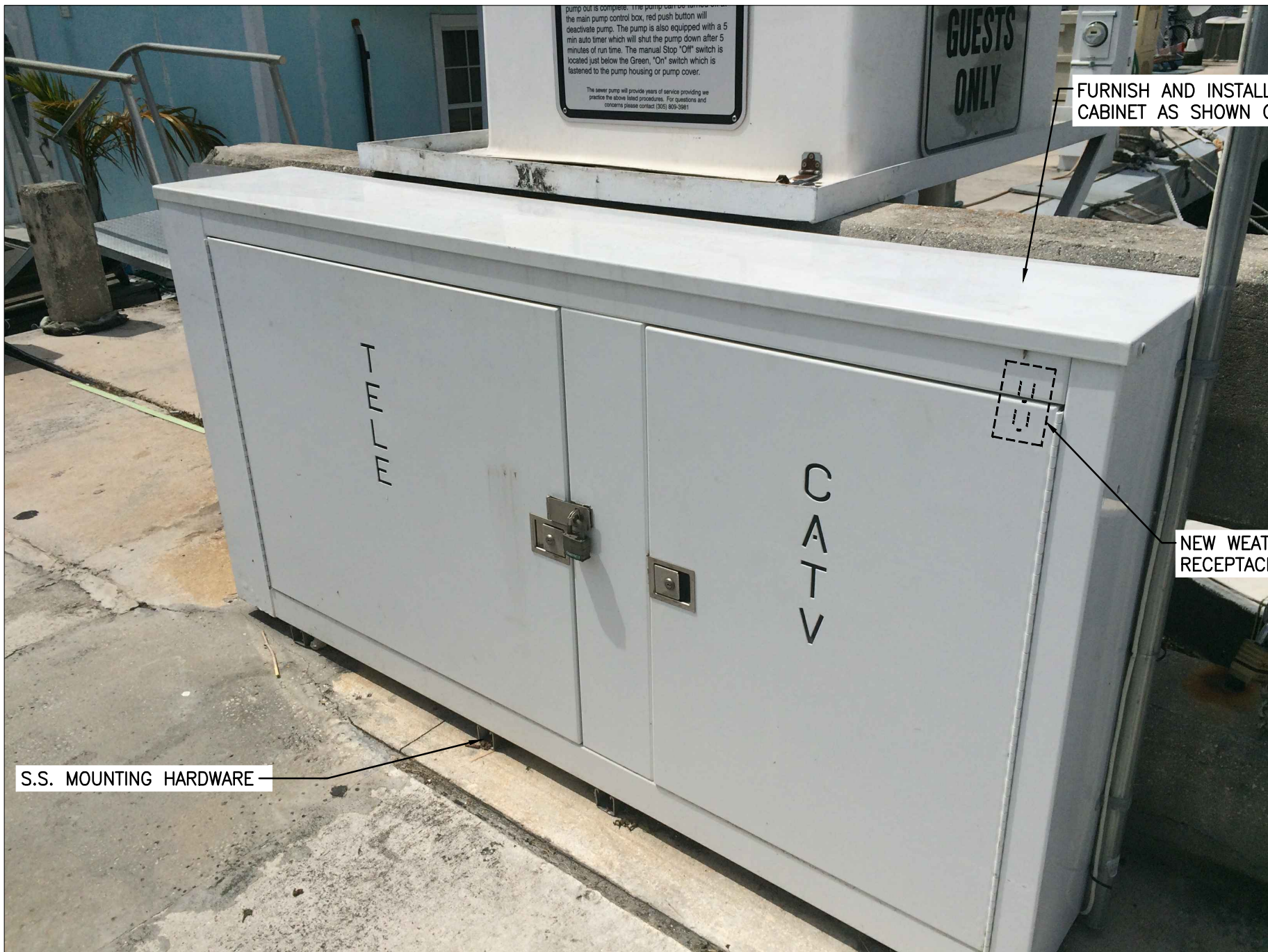
TELE/CATV CABINET DETAIL NO SCALE
