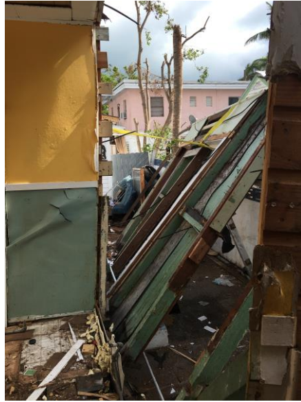
South Wall Crushed by Storm
