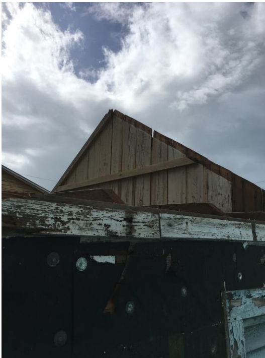
620 B Gable End Wall After Damaged Roof is Removed Note: 12/12 Pitch & 2' Knee wall at Upper Level Loft 14' Ht.
