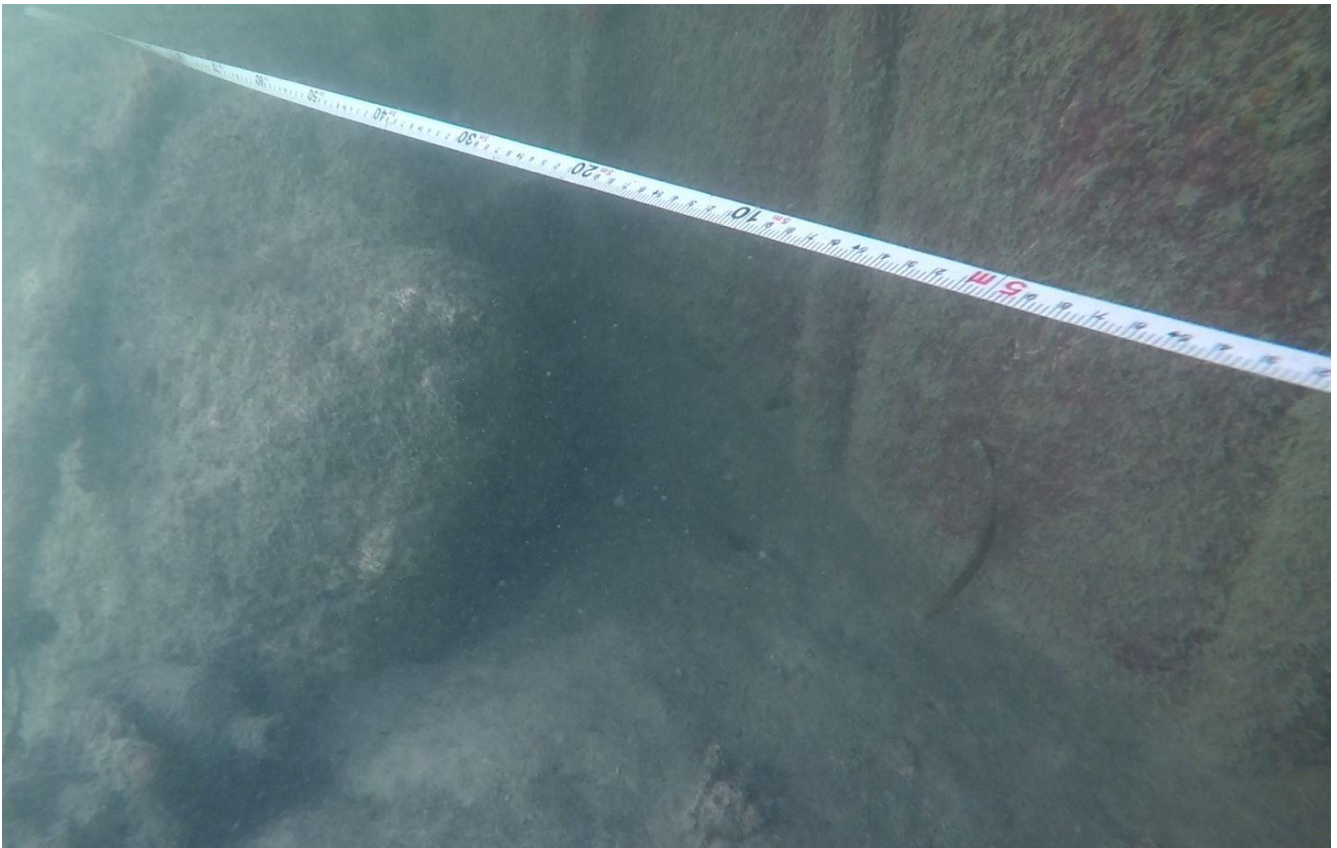
Underwater 5 - at 18ft 0in shows steel sheets driven through rock, rock sheered off left in front of wall
