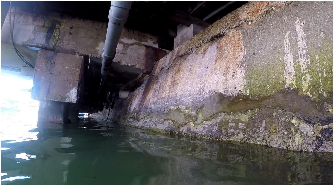
Underwater 17 - at 140ft above waterline looking east shows previous repairs and concrete piles supporting structures above wall
