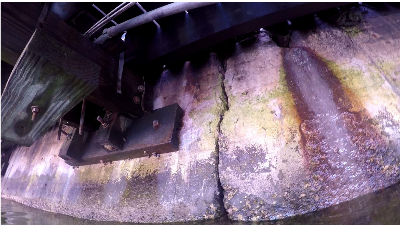
Underwater 32 - at 318ft above water shows large crack from top off wall all the way to the bottom
