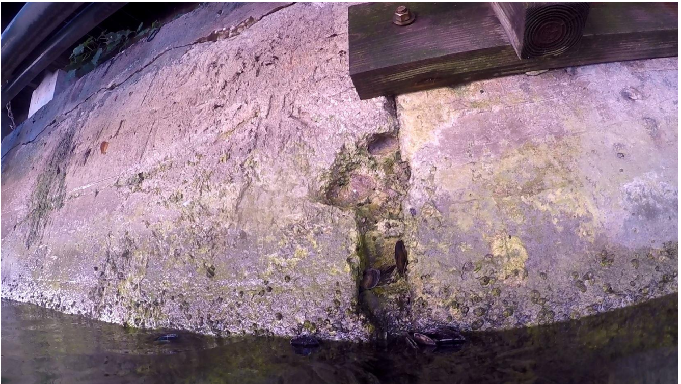
Underwater 24 - at 204ft shows old construction joint and spalling above the waterline
