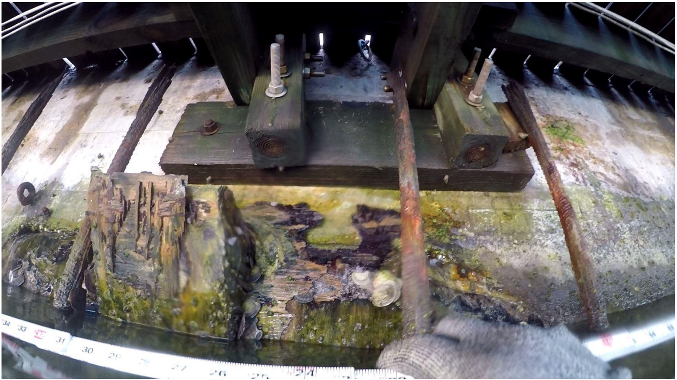
Underwater 35 - at 339ft shows a plug of some kind, with water leaking on both sides at top
