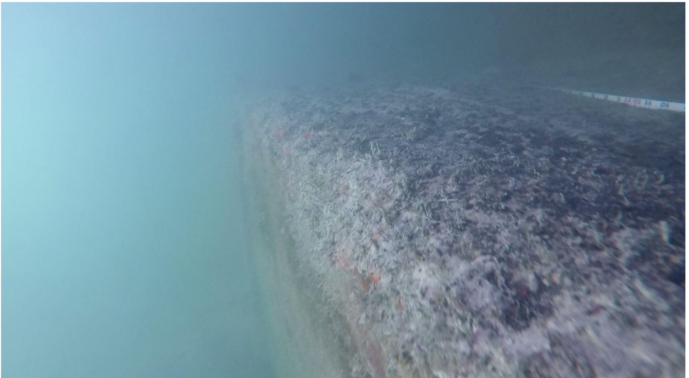
Underwater 11 - at 55ft shows concrete toe wall
