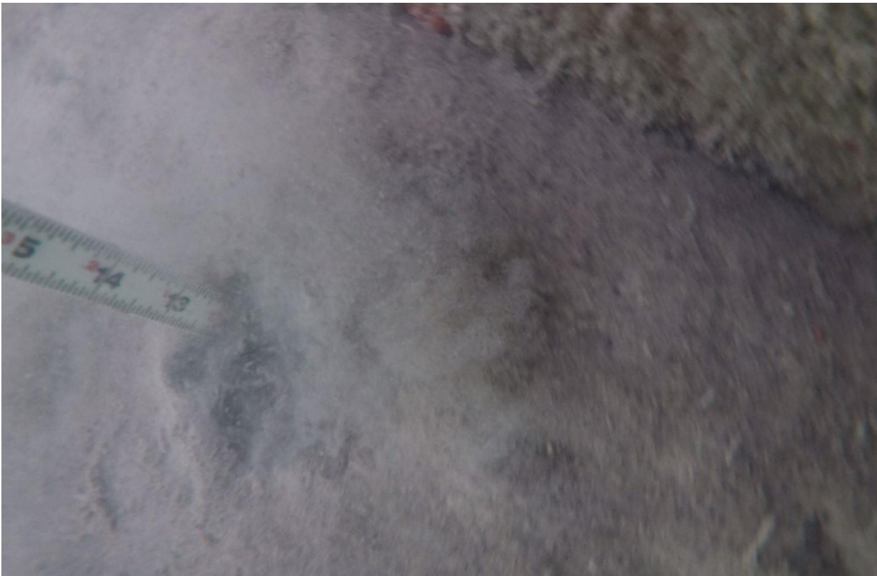
Underwater 15 - at 89ft shows sediment in front of toe wall 12in deep
