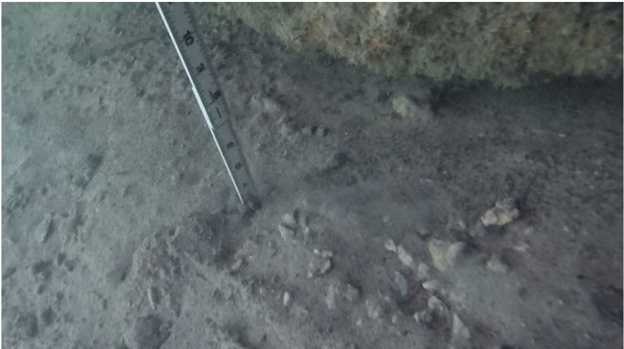
Underwater 2 - at 4ft 0in w continuous undermining at the toe and 4in sediment on top of rock
