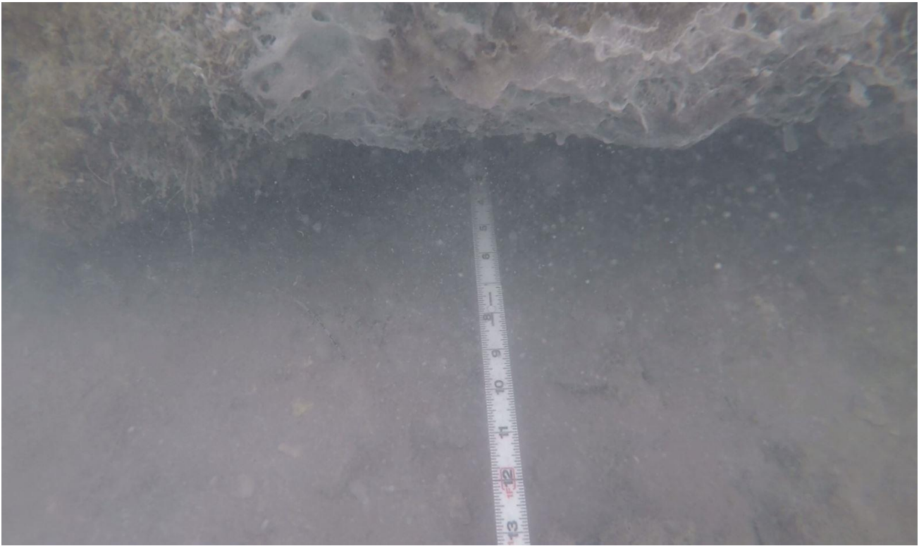
Underwater 27 - at 269ft shows 8in void at toe of wall
