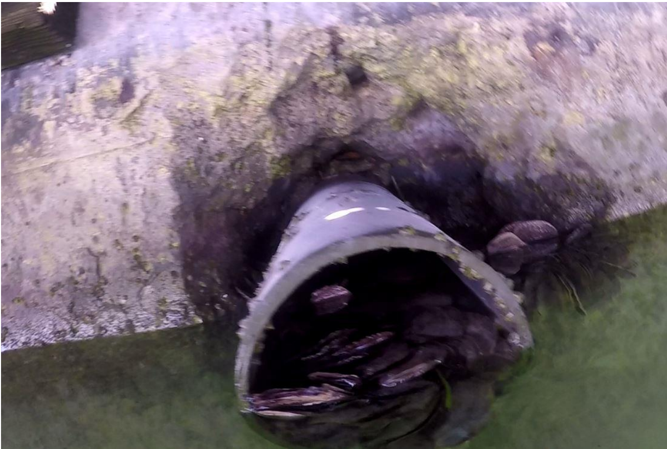
Underwater 28 - at 290ft above water line shows 12in diameter HDPE pile full of barnacles
