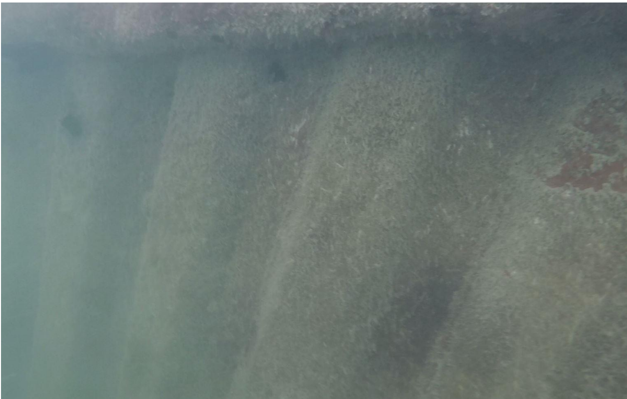
Underwater 16 - at 110ft shows steel sheet toe wall with concrete cap
