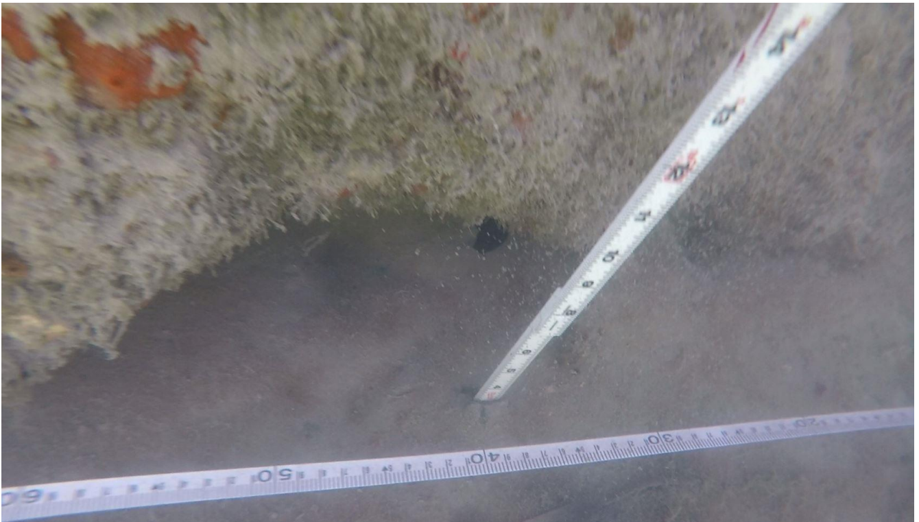
Underwater 40 - at 387ft showing 3in sediment in front of an 8in void
