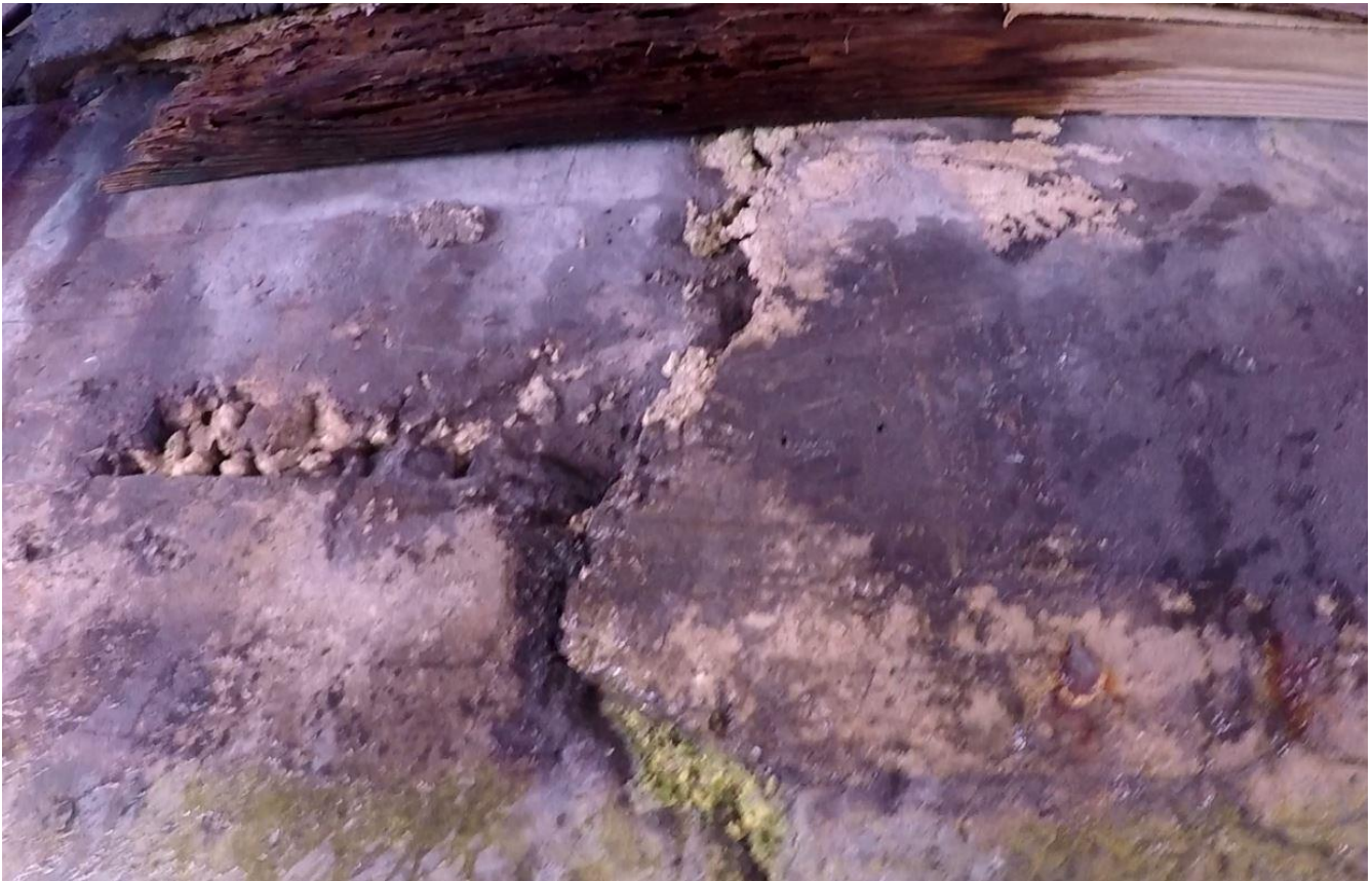
Underwater 20 - at 151ft above waterline shows large vertical crack
