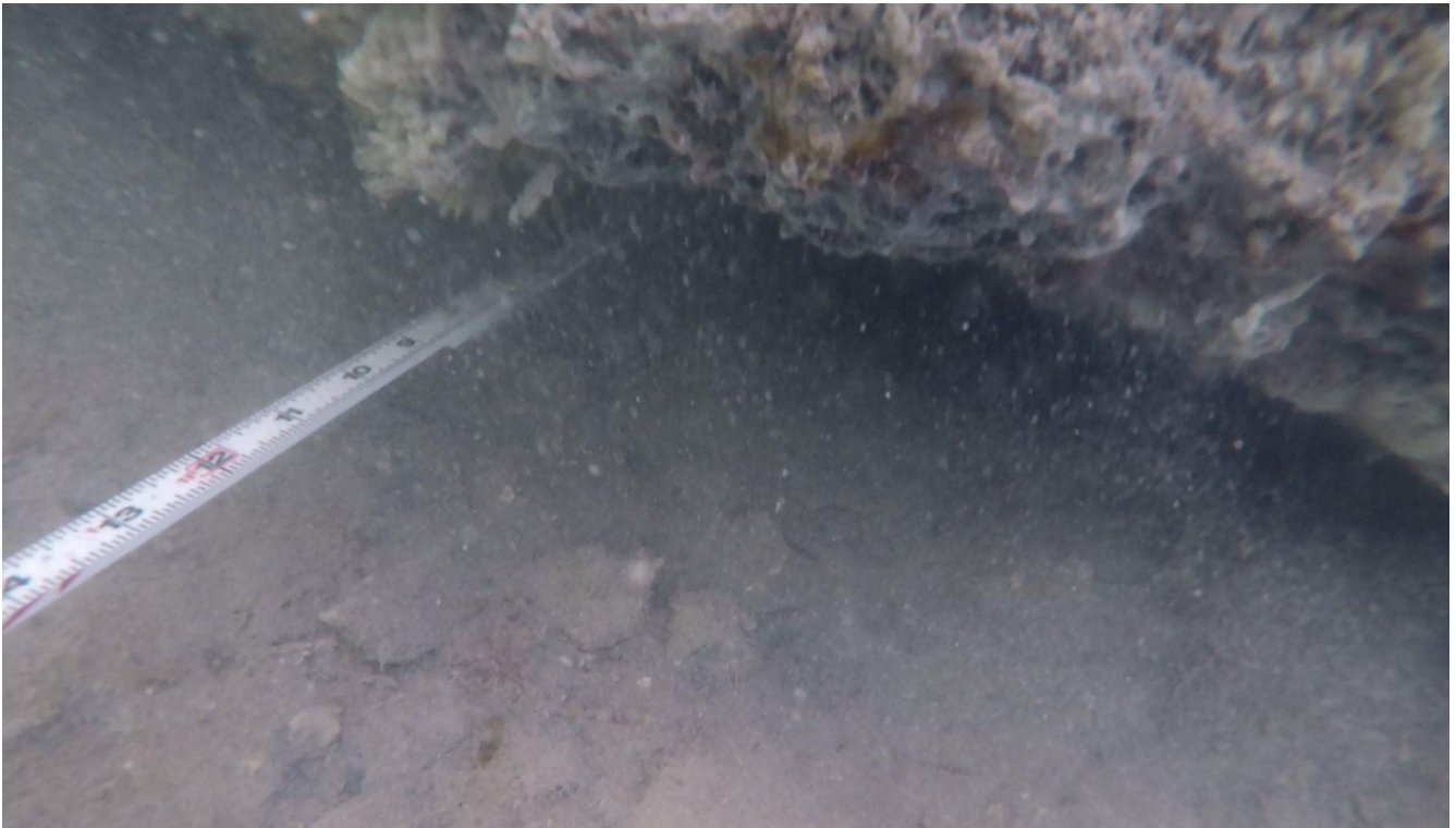
Underwater 25 - at 233ft shows 10ft long 8in deep void at toe of wall
