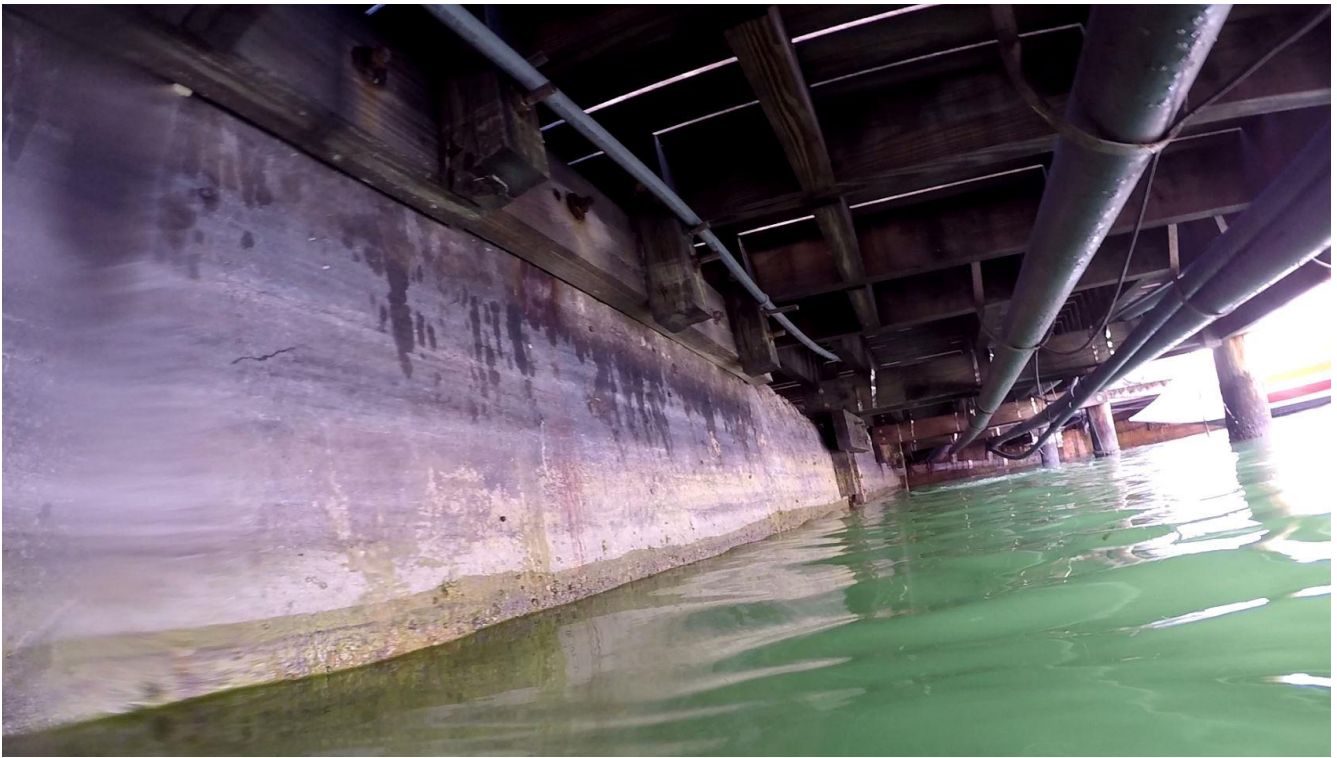
Underwater 9 - at 45ft above waterline looking west shows condition of concrete in good shape
