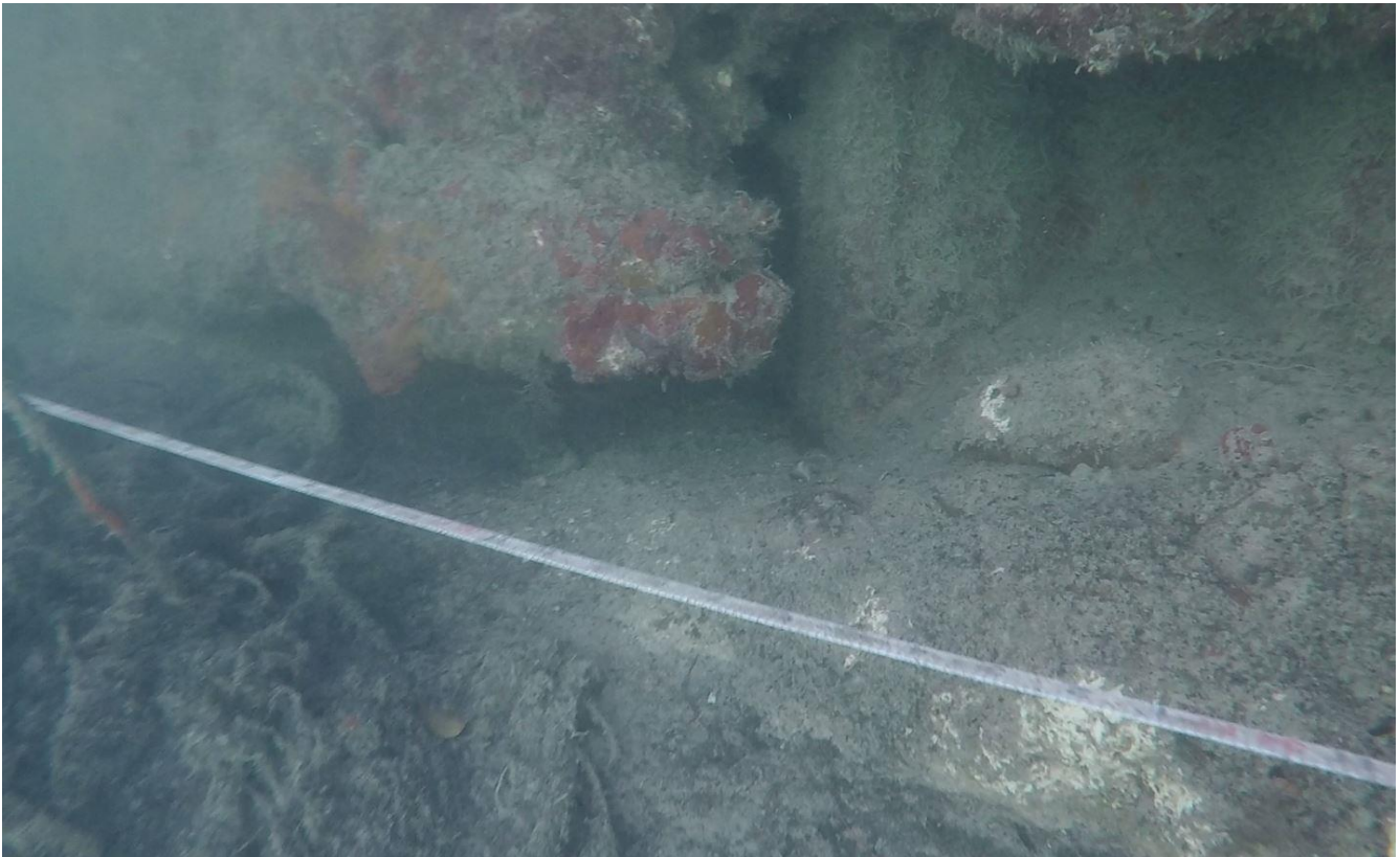
Underwater 6 - at 36ft steel sheet pile seems to have a void but it is only 6in deep at 36ft 8in
