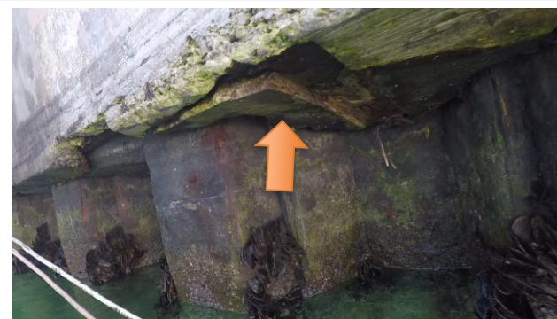
Figure 29: C-C, STA 1+57, Spalled cap
