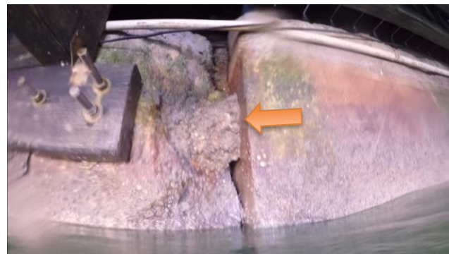
Figure 10: B-B, STA 0+50, Degraded Cold Joint
