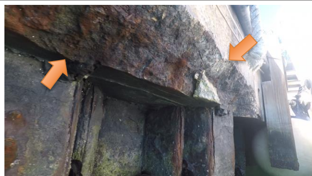
Figure 32: C-C, STA 1+90, Severely corroded cap
