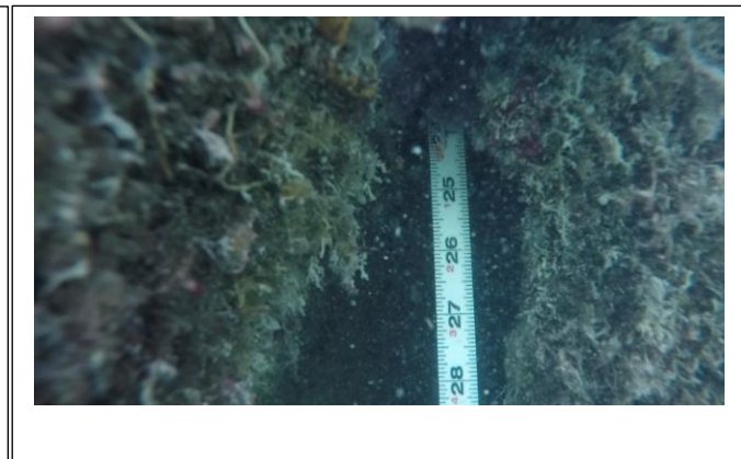
Figure 21: B-B, STA 2+86, Hole in sheet pile, 26" void
