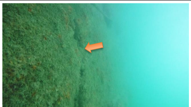
Figure 13: B-B, STA 0+87, Crack running below pipe
