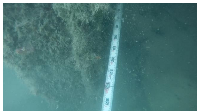
Figure 28: C-C, STA 1+36, Void space of 20"
