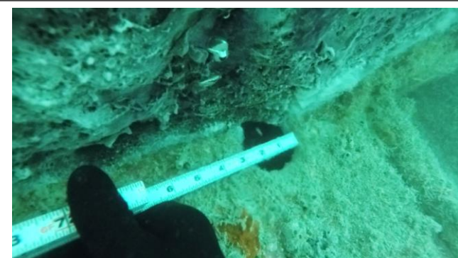
Figure 15: B-B, STA 1+00, Ficus roots overhang wall
