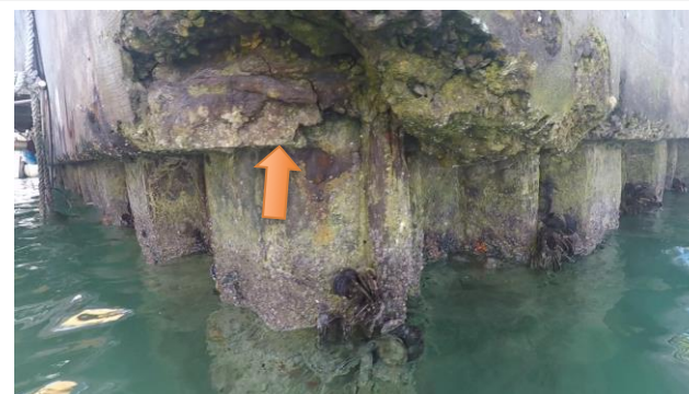
Figure 33: C-C, STA 2+55, Large spalling area
