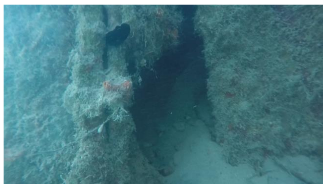
Figure 26: C-C, STA 1+36, Separation of sheets (View 1)
