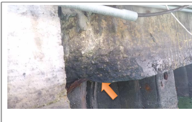
Figure 23: C-C, STA 0+57, Spalling cap
