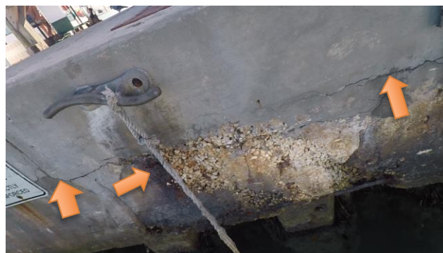
Figure 35: D-D, STA 0+10, Honeycomb with cracks
