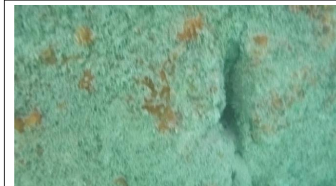
Figure 12: B-B, STA 0+87, Pipe Penetration w/ Cracking
