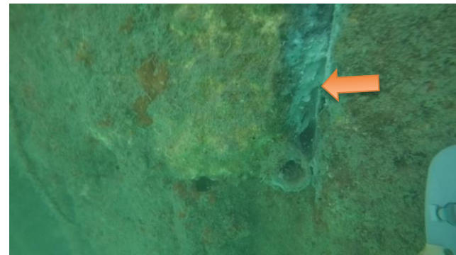
Figure 11: B-B, STA 0+50, Degraded Cold Joint
