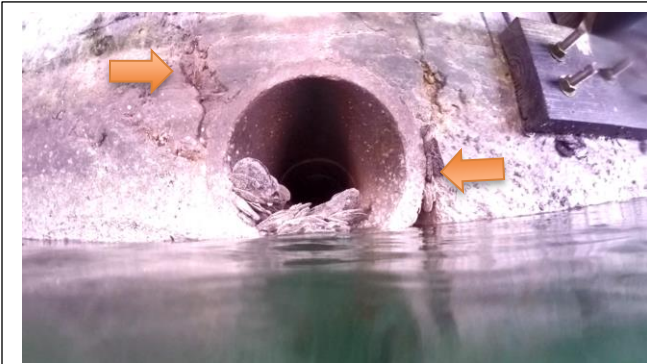
Figure 12: B-B, STA 0+87, Pipe Penetration w/ Cracking
