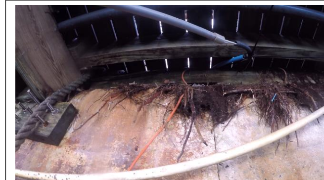
Figure 14: B-B, STA 0+87, Split, spalled joint beneath pipe
