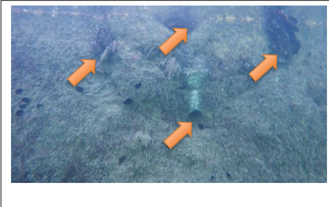
Figure 18: B-B, STA 1+71, Several 3" Dia. holes in cap
