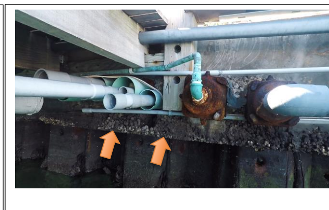
Figure 25: C-C, STA 0+65, Honeycombing in cap
