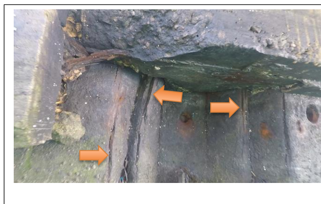
Figure 24: C-C, STA 0+57, Severely corroded sheets
