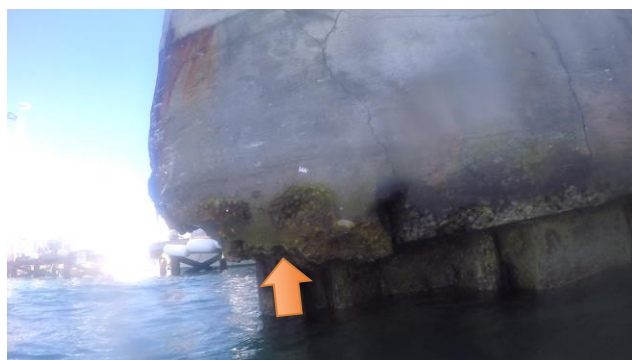
Figure 34: D-D, STA 0+00, Spalled cap at corner
