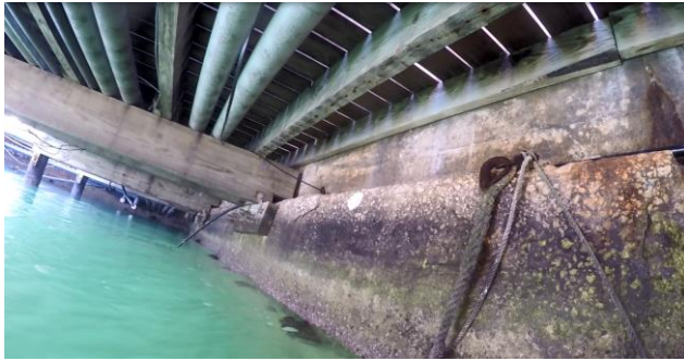
Figure 8: B-B, STA 0+00, Representative example of pitting
