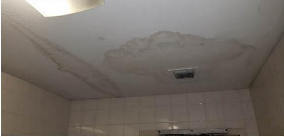
Figure 23. Water damage to the drywall ceiling in the front section of the building in the bathroom. (likely prior new roofing installation). Please note that all locations were dry during the inspections – however no recent significant rain events.
