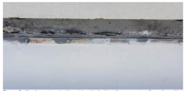
Figure 8. Membrane termination strip attached to the parapet walls and cracking sealant. No protective flushing is installed over the termination strip. Failure of the sealant will likely result in water intrusion into building envelope.
