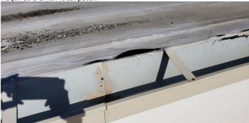
Figure 10. Pealing up edge of the membrane at the gutter between two roof levels. Requires maintenance.
