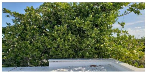
Figure 5. Same new roofing with tree branches overhanging and tree debris collecting along the short parapet walls. All trees around the building should be professionally pruned to prevent damage to the roofing and structure cladding.
