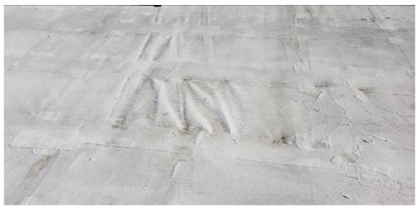
Figure 6. Aging membrane surface with adhesion imperfections, small patches and liquid applied coating. Page 5  $_{\text{DF}}$  27
