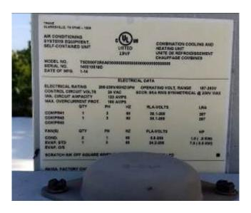
Figures 27&28. Rooftop package unit servicing front of the building. Trane Voyager Model# TSD300F3R0A030, Date of Manufacturing 1-14. 25 Tons Standard Efficiency, 208-230/60/3 phase.
