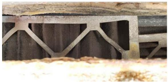
Figure 29. Dirty fresh air intake filters are visible through the otherwise unprotected opening. Requires maintenance and coil cleaning.
