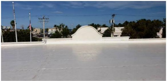
Figure 3. View over new roofing membrane vinyl (TPO) over tapered insulation. Roofing surface looks good, small imperfections reflect uneven nature of the underlaying insulation capping sheet. The roofing is likely to be under current construction warranty and manufacturer material warranty. Owner should be contacted directly to transfer all warranties as part of the closing procedures if the City decides to proceed with the purchase.
