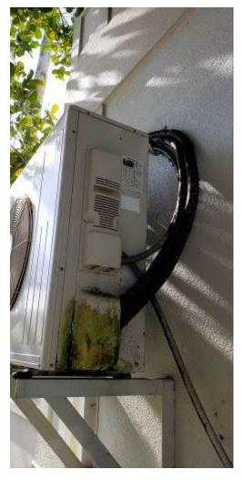
Figures 32&33. Minisplit unit servicing IT Server room (East Side of the building). Line insulation excessive sweating and waterlogging. The unit requires maintenance, all lines insulation needs to be replaced, coils cleaned, and refrigerant levels checked.
