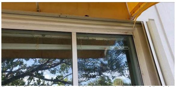
Figure 21. Signs of water intrusion – visible damage to the drywall trim of the window opening on the interior (likely prior new roofing installation).
