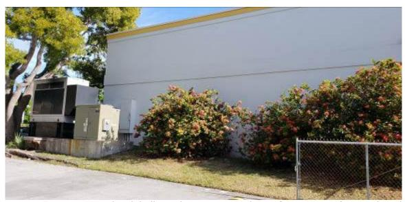
Figure 35. Concrete pad with belly-tank generator and transformer. Transfer switch and disconnect on the building wall behind.
