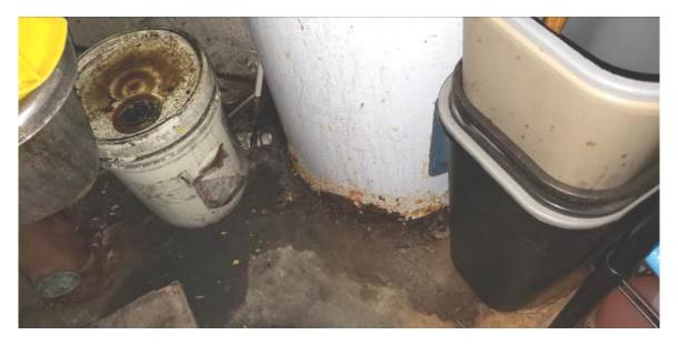
Figure 40&41. Hot water tank. Functional but will require replacement due to corrosion of the outer shell.
