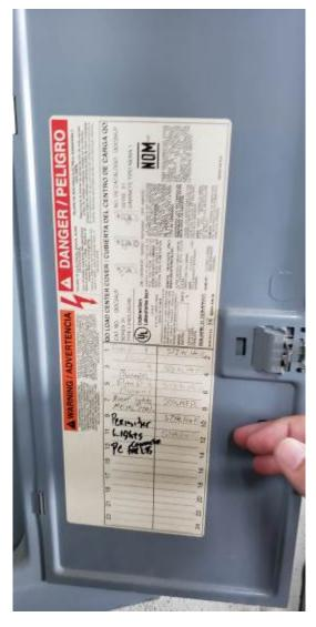
Figures 37&38. Multiple load centers are installed in various locations inside of the building with local brokers for lights, receptacles and various printing equipment. The condition of the electrical systems is good and serviceable.
