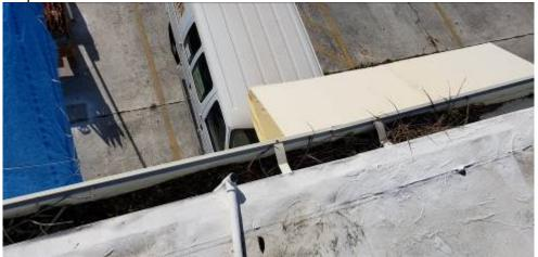
Figure 11. Tree leaves and branches in the rear gutter, requires maintenance, tree pruning and perhaps leaf guard for the gutter system.
