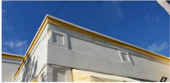
Figure 13. Exterior wall with small damage to the corner and surface (likely hurricane debris damage). Similar small damage in other locations. Cosmetic repairs are needed.
