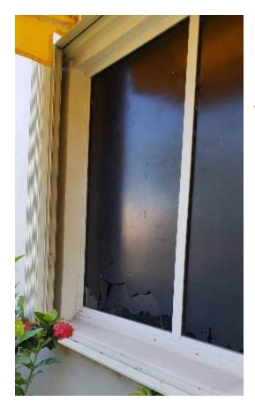
Figure 18. Broken outer pane of a double glass fenestration system in one location. Replacement of the glass is needed. Please note that some windows have black-out coating for privacy.
