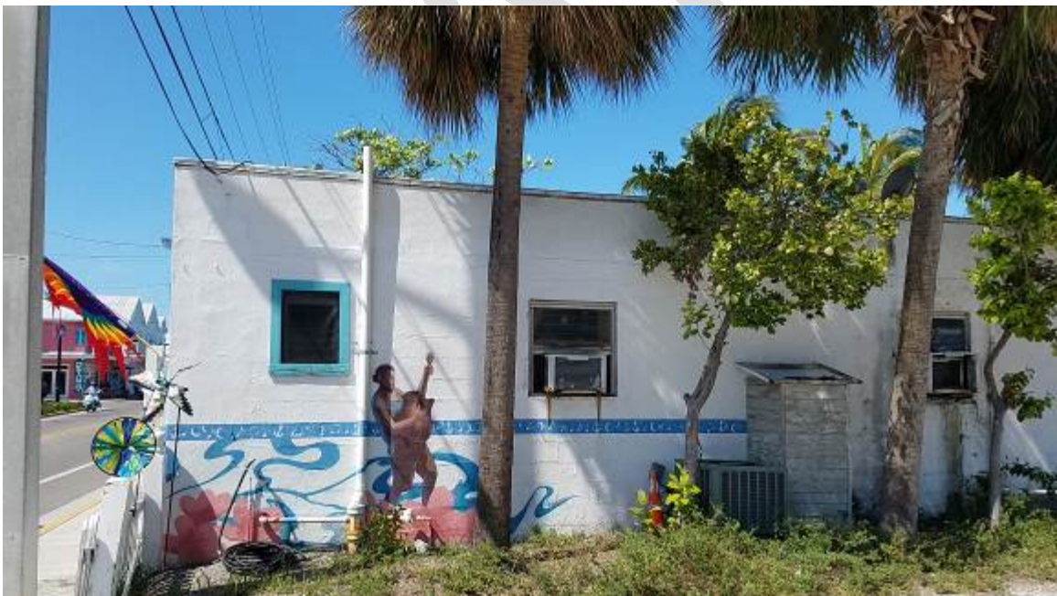
Figure 4. Partial right side elevation. More cracks in the tie-beam. Damaged jalousie style glazing with window a/c units.
