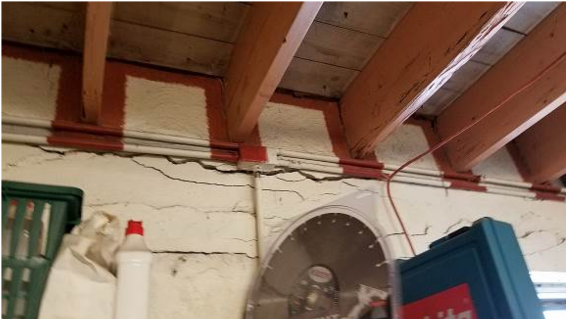
Figure 11. Same as above. Heavy concrete damage, damaged rafters and more electrical conduits.
