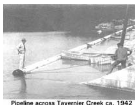
Pipeline across Tavernier Creek ca. 1942
