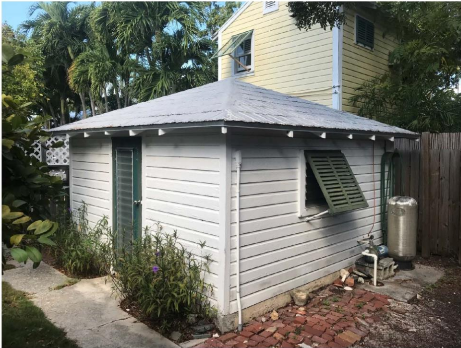
1227 WASHINGTON STREET REAR POOL HOUSE FRONT/SIDE VIEW
