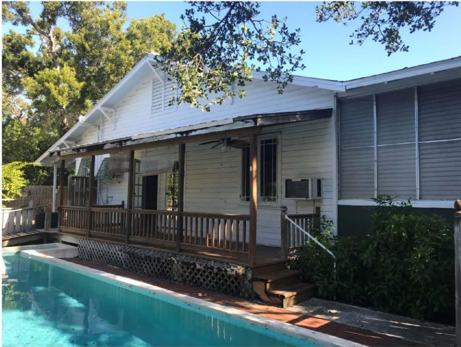
1227 WASHINGTON STREET SIDE VIEW
