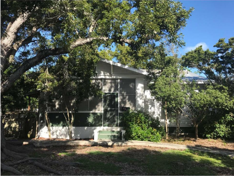
1227 WASHINGTON STREET FRONT VIEW
