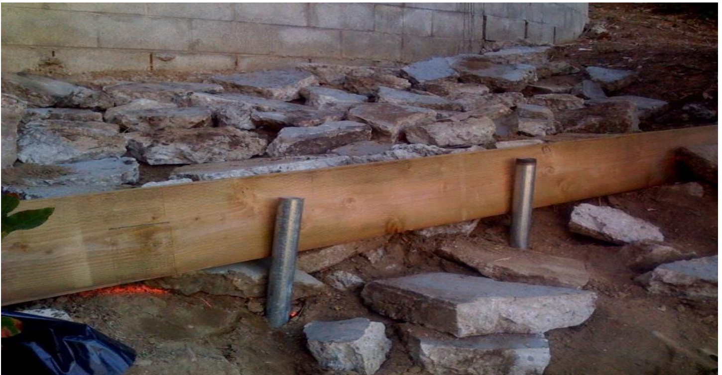
Micro Retaining Walls Rebar for RWS
