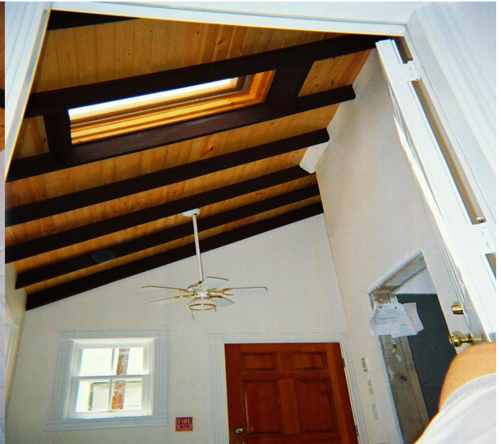
NEW MANAGERS OFFICE WITH VELUX RAIN AUTO-CLOSE HATCHES
