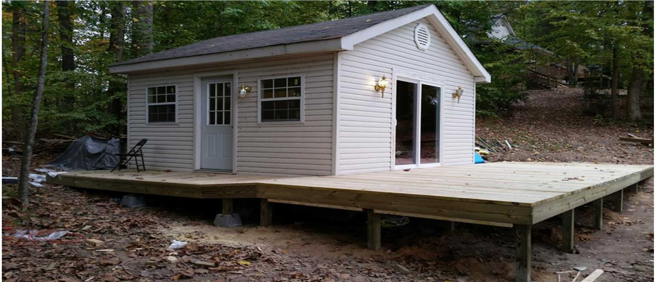
FOUNDATION BAD DESIGN AND CONSTRUCTION
