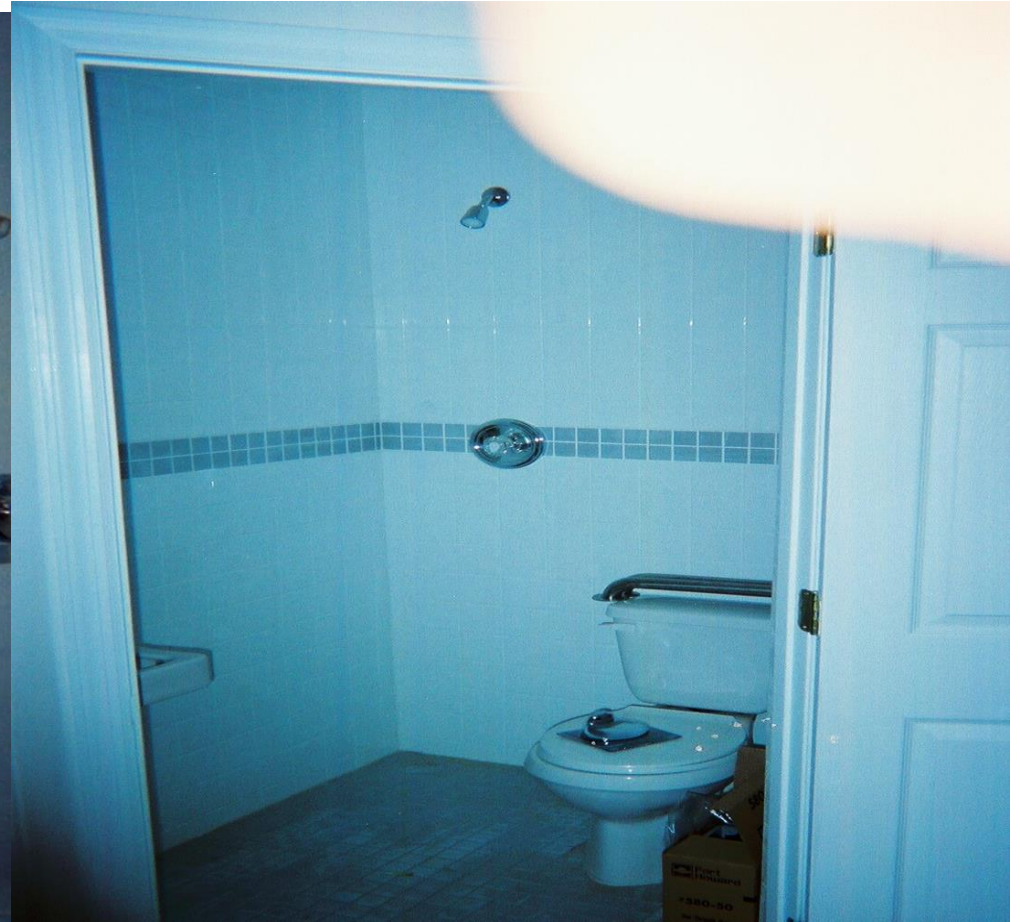
FULLY TILED BATHROOM WITH FLOOR DRAIN IS 4' X 5' TOILET/ SHOWER
