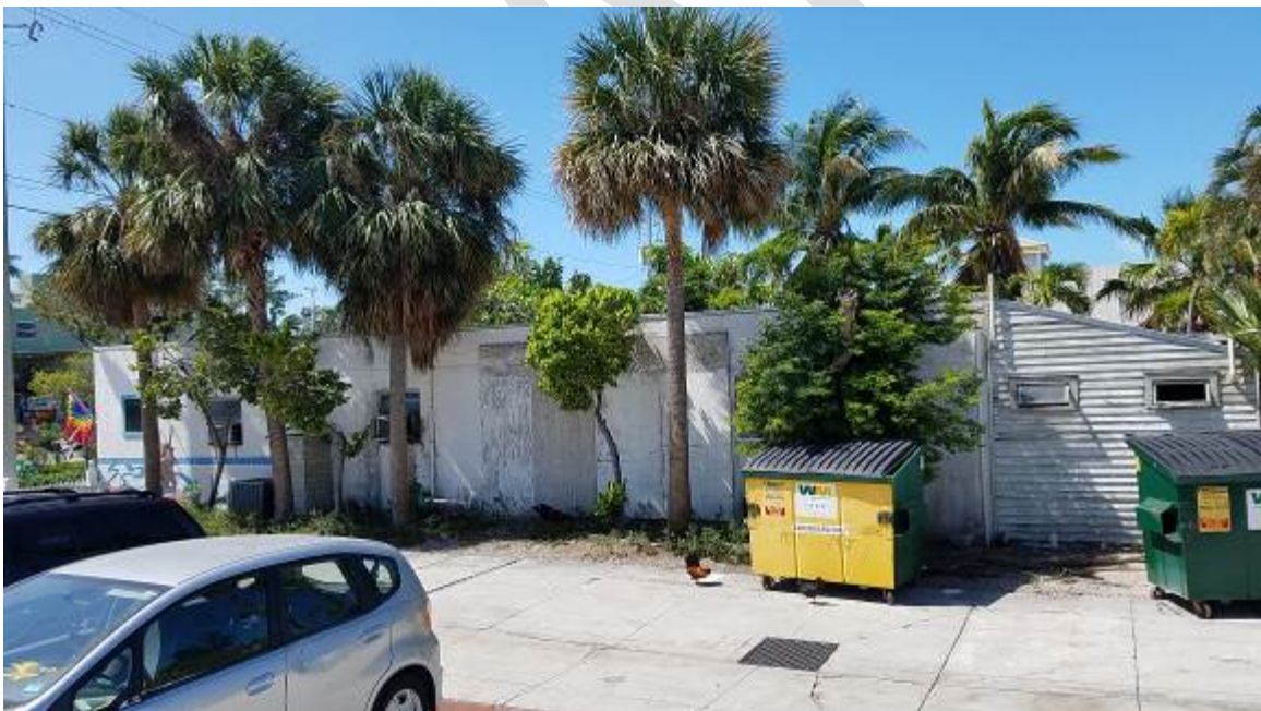
Figure 8. Overall right side elevation with rear wood frame shed.
