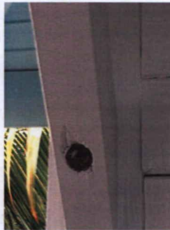
(Pic. 11) Upstairs bar wood bracing (Missing bolt connector)
