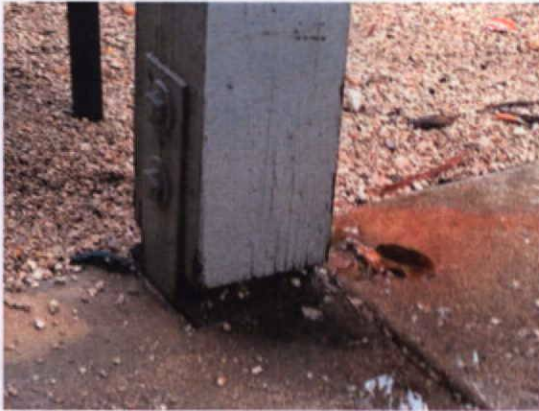
(Pic.6) Wood column post at covered walkway (Gap at base)
