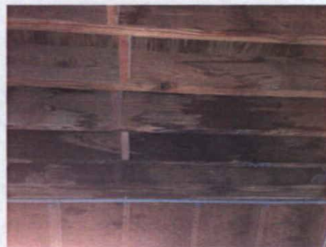
(Pic.5) Typical Roof Framing Weathered & Wet from Moisture Intrusion
