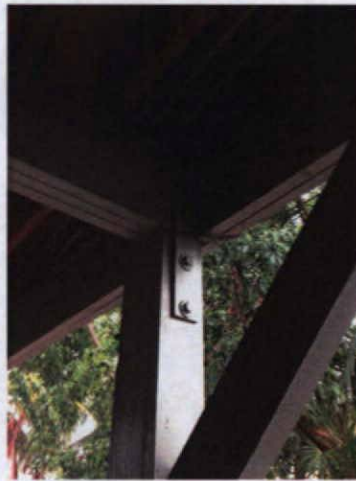
(Pic.3) Typical Perimeter Roof Support
