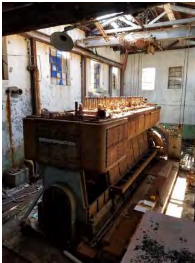
Nordberg Dynamo generator in Building 4
