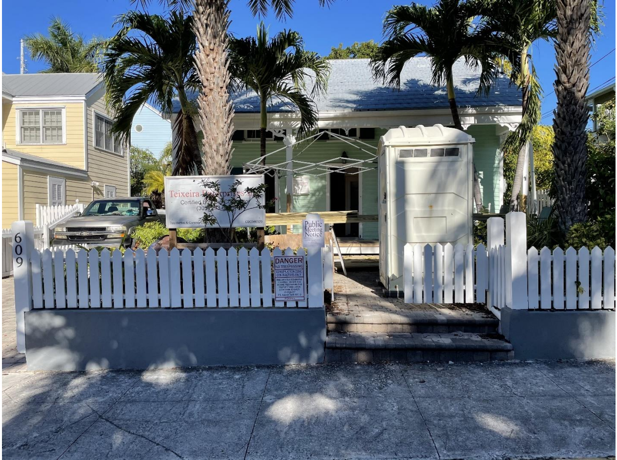
Photo one of notice posted at 609 Angela Street.
